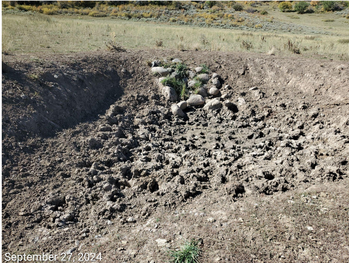
Photo 6: Sediment trap/drain on south end of the well pad Location.
