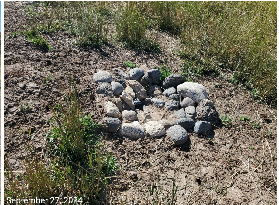
Photo 3: Sediment trap / drain on the southwest corner of the battery facility pad.
