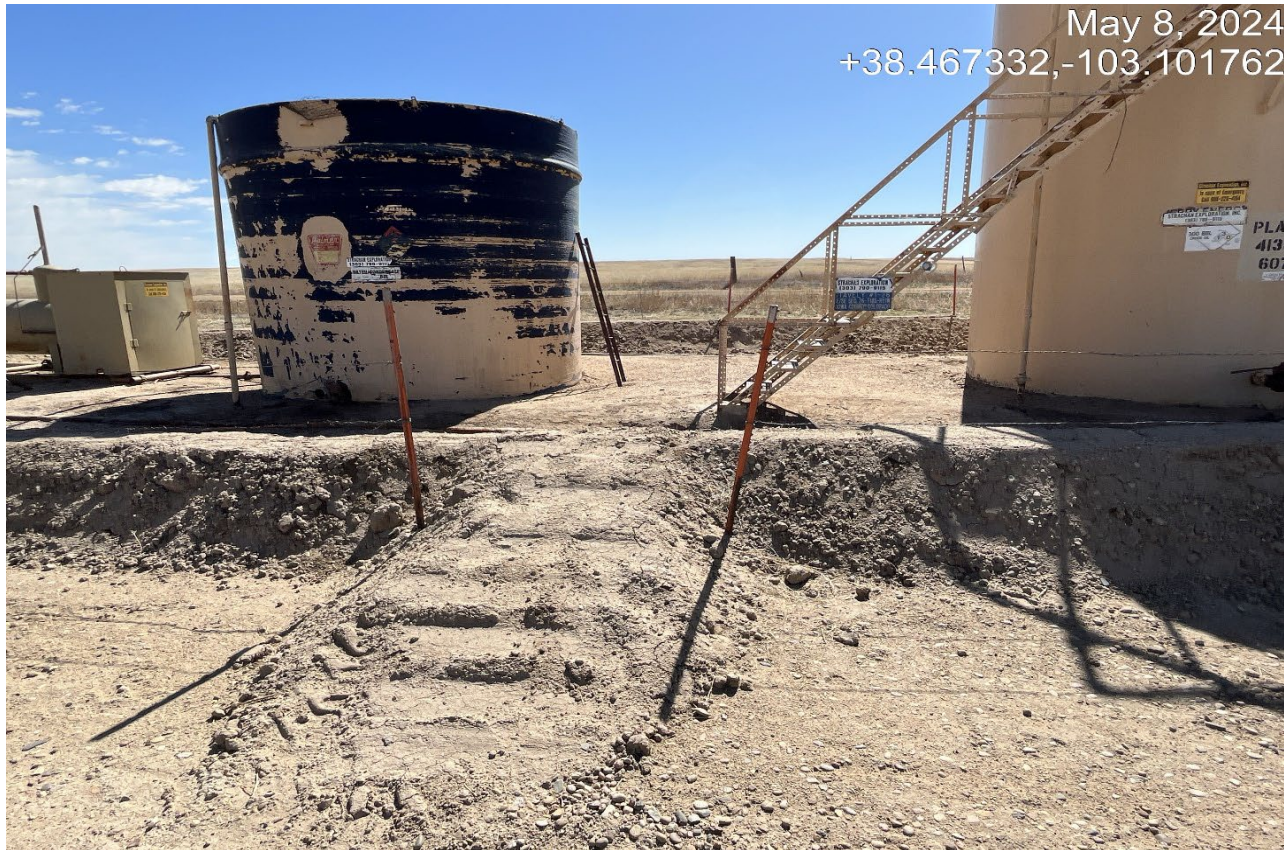
Photo 2. The fence around the tank has been repaired but there is an opening at this area and there are only 2 wires which will not keep livestock out.
