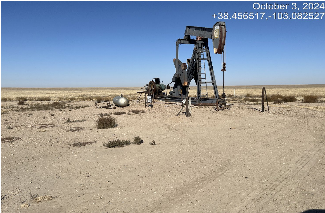
Photo 3. Facing northwest toward the wellsite. The fence around the pumpjack is in disrepair and wont prevent livestock entry. A new well sign has been installed.
