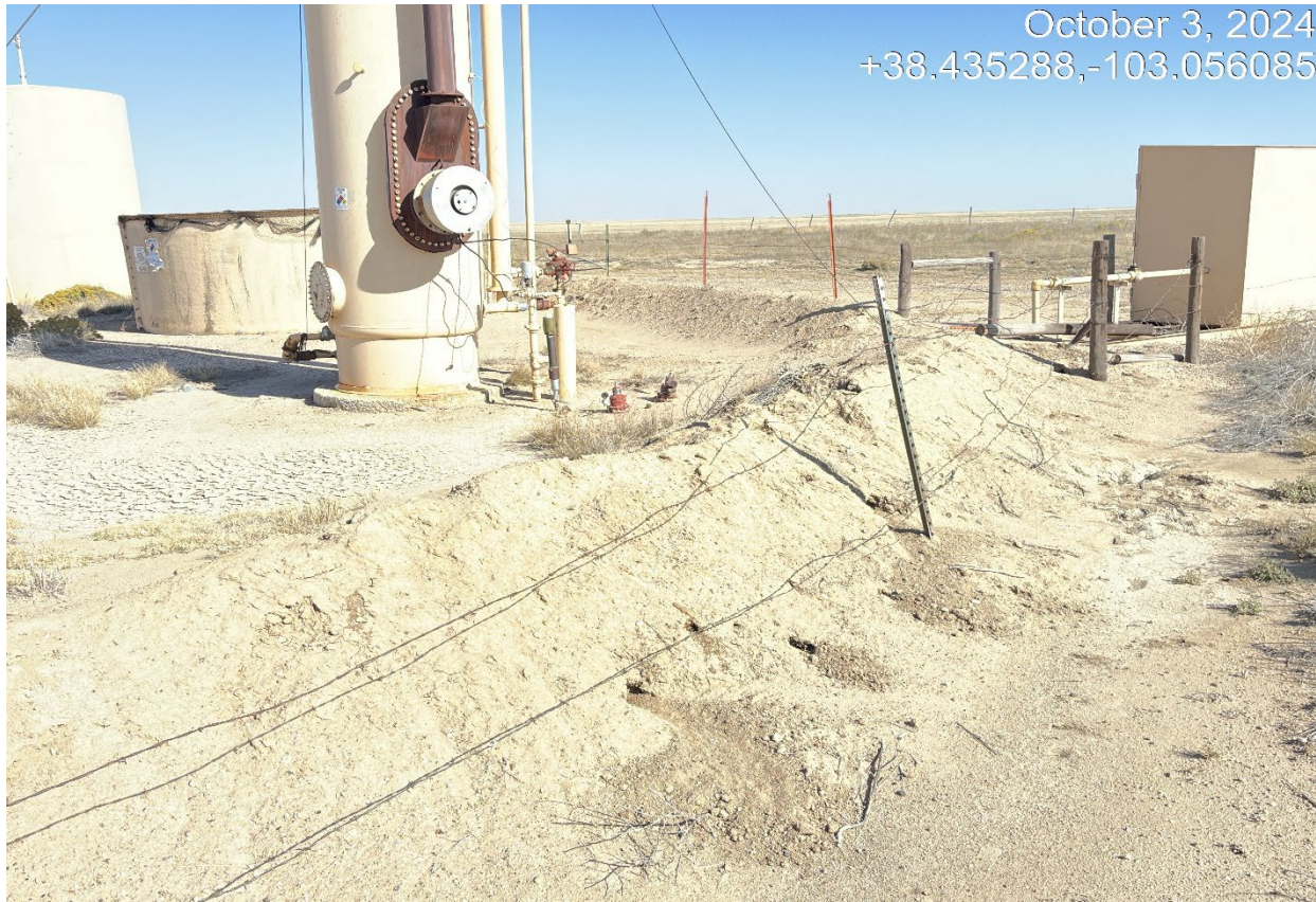
Photo 4. The 2 strand fence is inadequate to prevent livestock entry. Previous CA was not completed.
