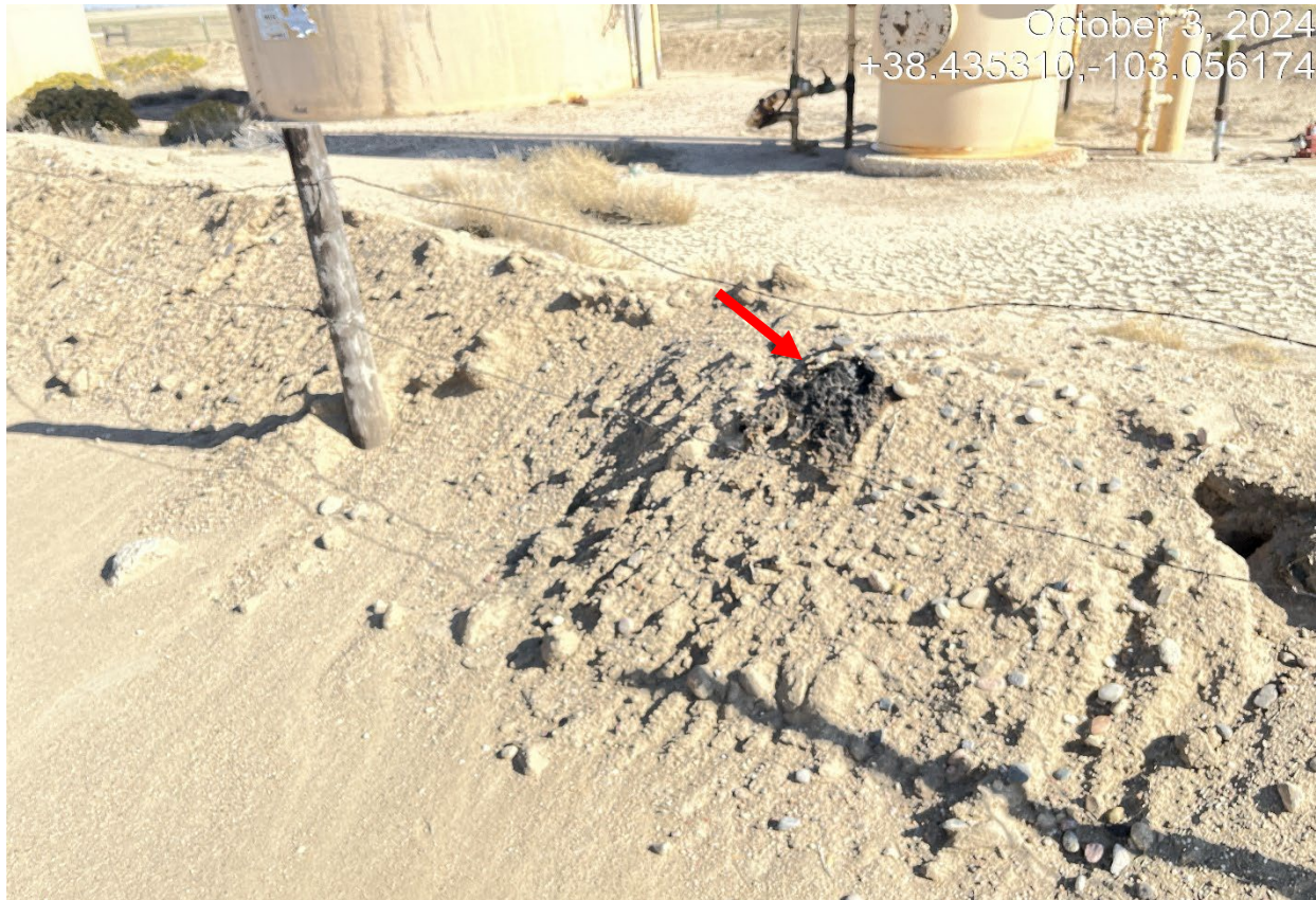
Photo 3. There is oily sludge on the berm that needs to be cleaned up.
