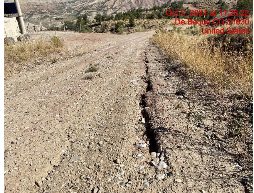
Rill Erosion on Lease Road – Photo #03937
