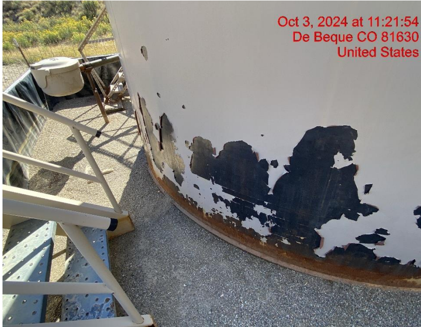
Paint is Peeling From Tank – Photo #03932
