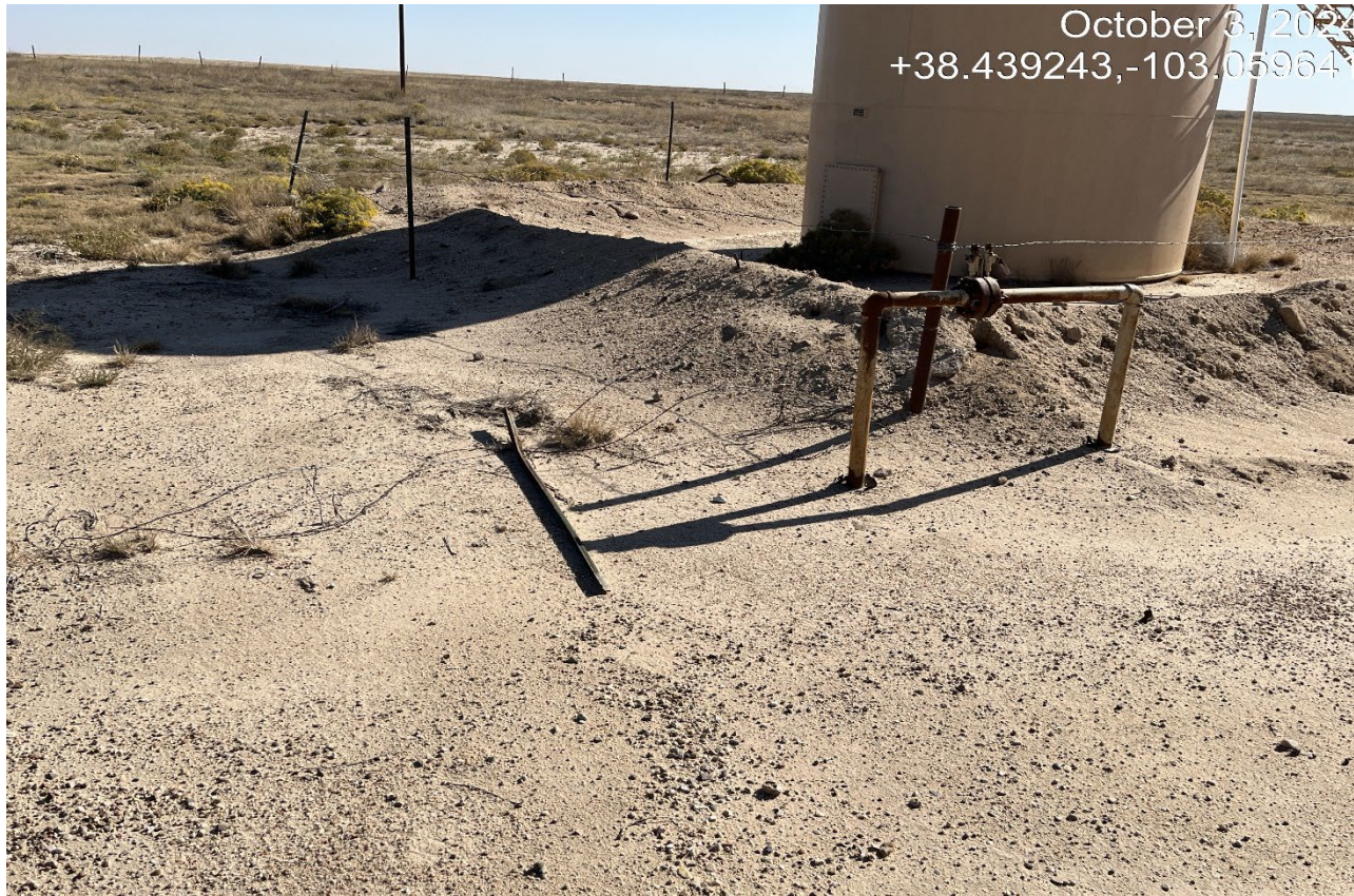
Photo 14. Facing at the north side of the location. The fence around the tank battery is inadequate to prevent livestock entry and is not maintained. The berm around the tank has been rebuilt.
