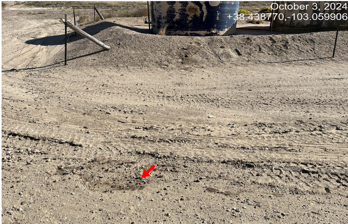
Photo 8. Facing northeast by the tank battery. There is still oil stained soils where spill crude oil was spread along the road. Red arrows point to visible oil impacted soils.
