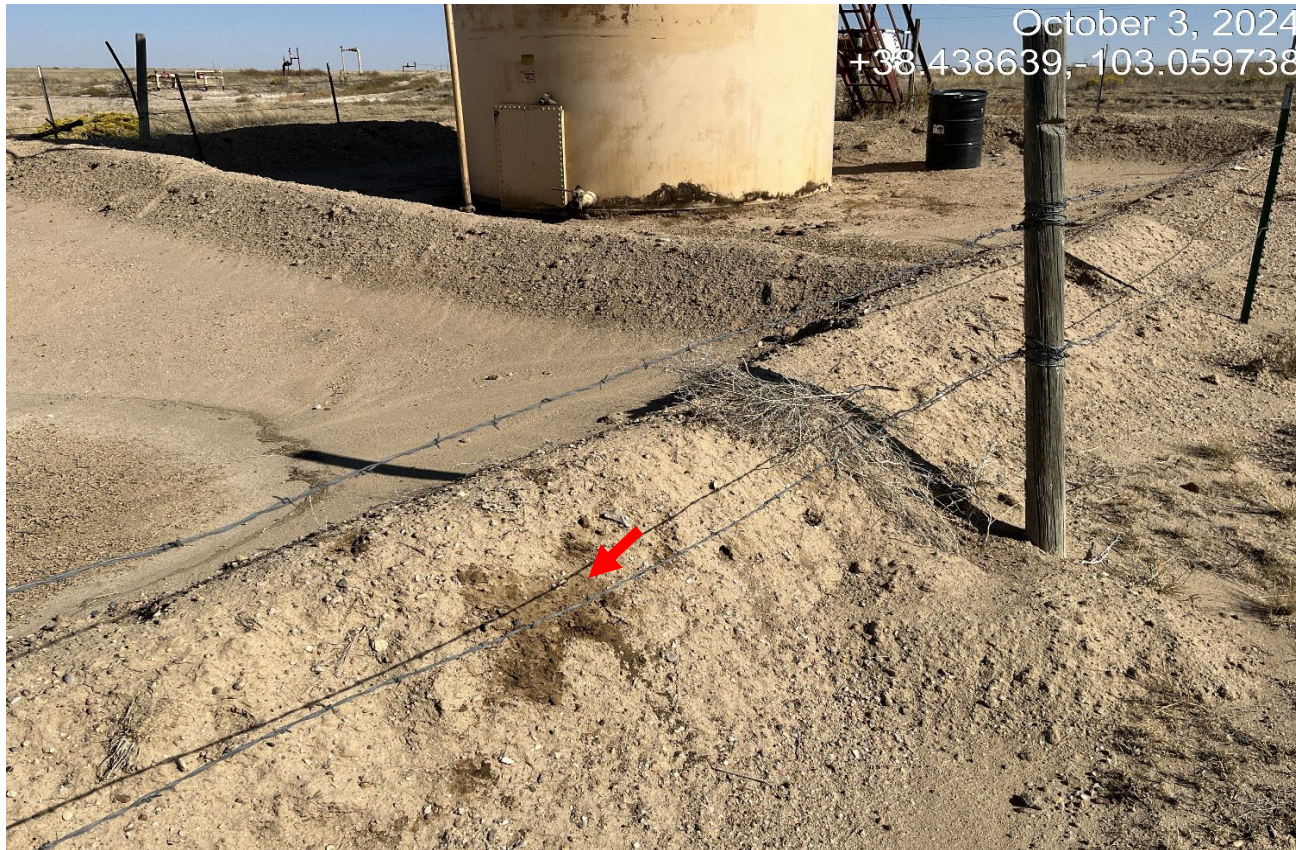
Photo 10. The berm around the tanks has been rebuilt but contains oily impacted material with hydrocarbon odor. The contaminated berm material must be removed and properly disposed. Previous CA was not completed.
