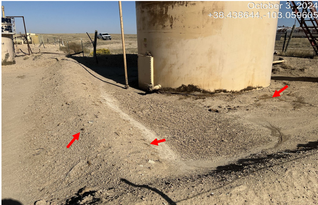
Photo 11. The berms around the tanks contains oily impacted material with hydrocarbon odor. The spill at the tank has not been cleaned up. Previous CA was not completed.
