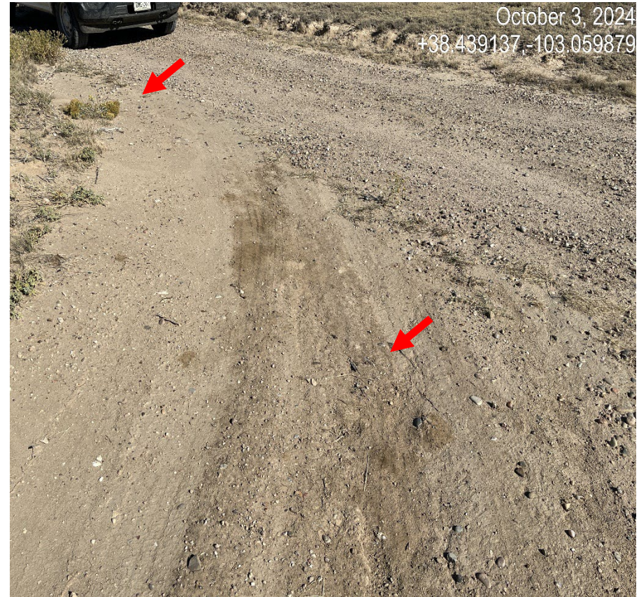
Photo 4. View of the stained soils that still remains along the road where oily material was spread along the road.
