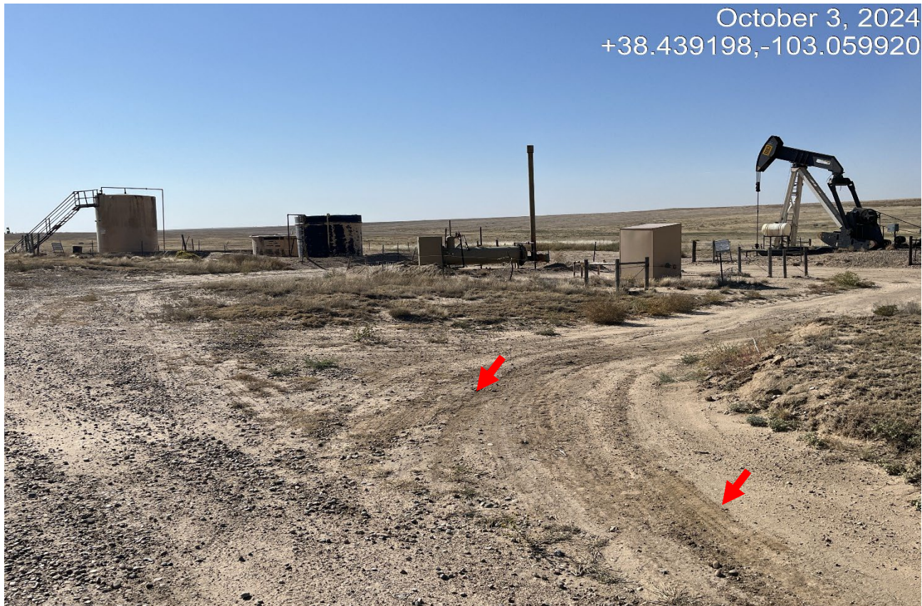
Photo 2. Facing southeast toward by the wellsite. Impacted oily soils was spread all the way from the tank battery to the roadway. Red arrows point to visible impacted stained soils that have not been cleaned up. Previous CA was not completed.
