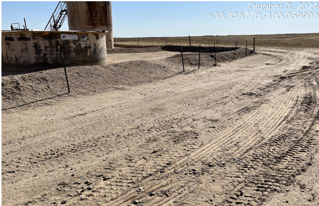
Photo 9. Facing northeast toward the tank battery where previous spill had occurred. The berm around the tanks has been rebuilt but contains oily impacted material with hydrocarbon odor.
