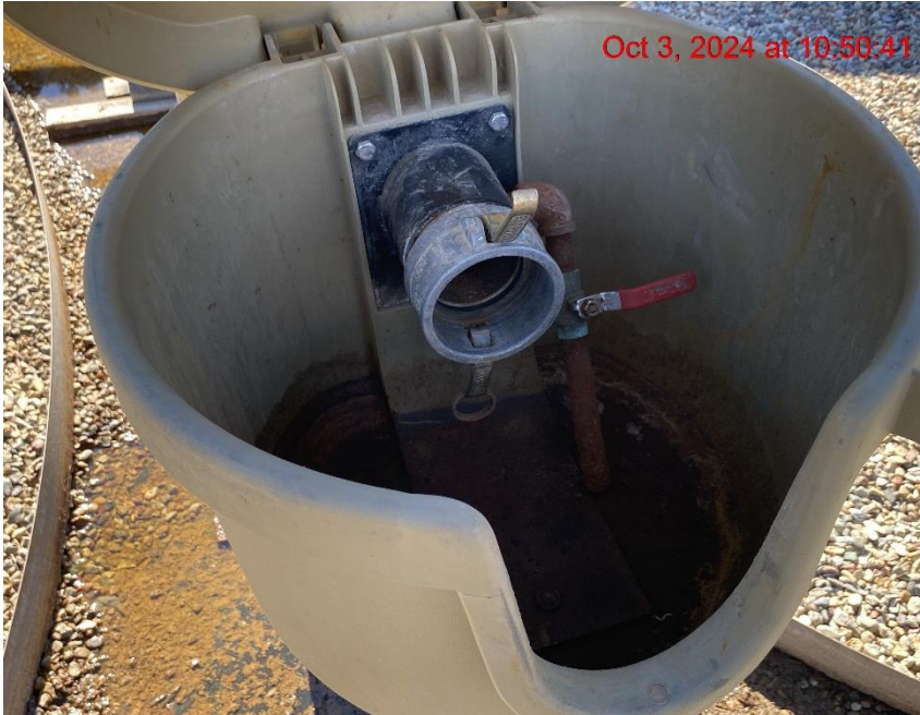
Open-Ended Load Line – Photo #03890
