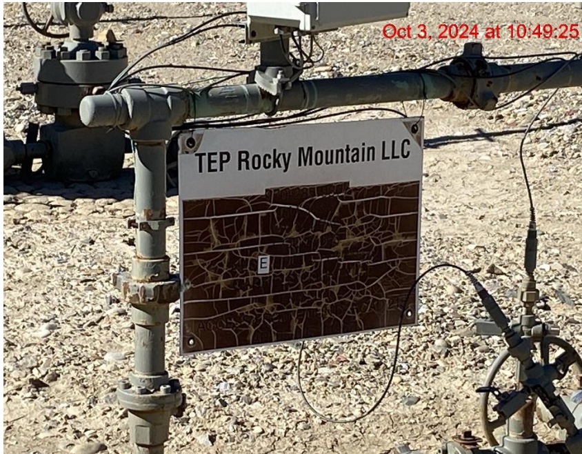
Weathered and Illegible Wellhead Sign – Photo #03886
