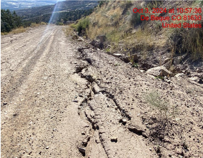
Insufficient Erosion Control; Rill Erosion on Lease Road – Photo #03900
