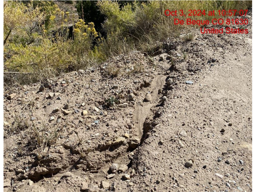
Insufficient Erosion Control; Transport of Sediment Off of Lease Road – Photo #03898
