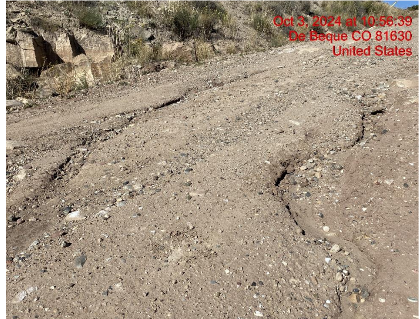
Insufficient Erosion Control; Rill Erosion on Lease Road – Photo #03896
