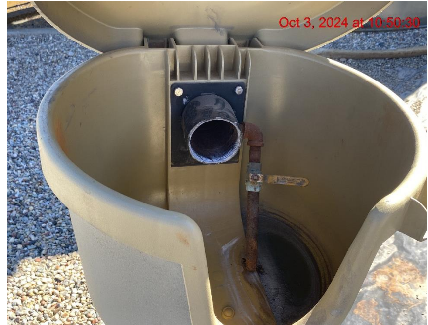
Open-Ended Load Line – Photo #03889
