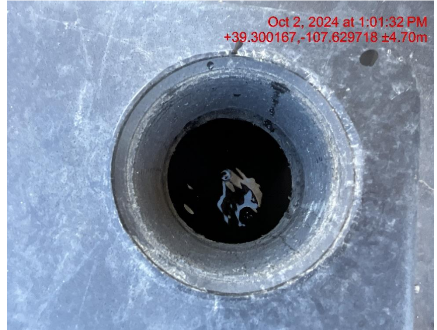
Failure to maintain chemical BMP/chemical tank containment ¾ full of fluid - Photo #06972
