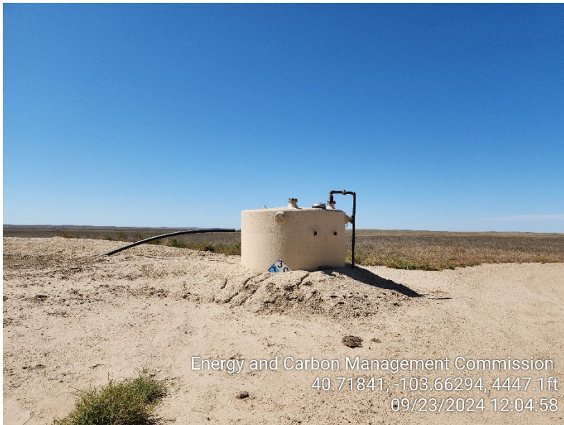
Photo 7 – Skim Tank – Missing Tank Labels
