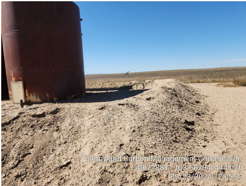
Photo 11 – Tank Battery – Berms Inadequate
