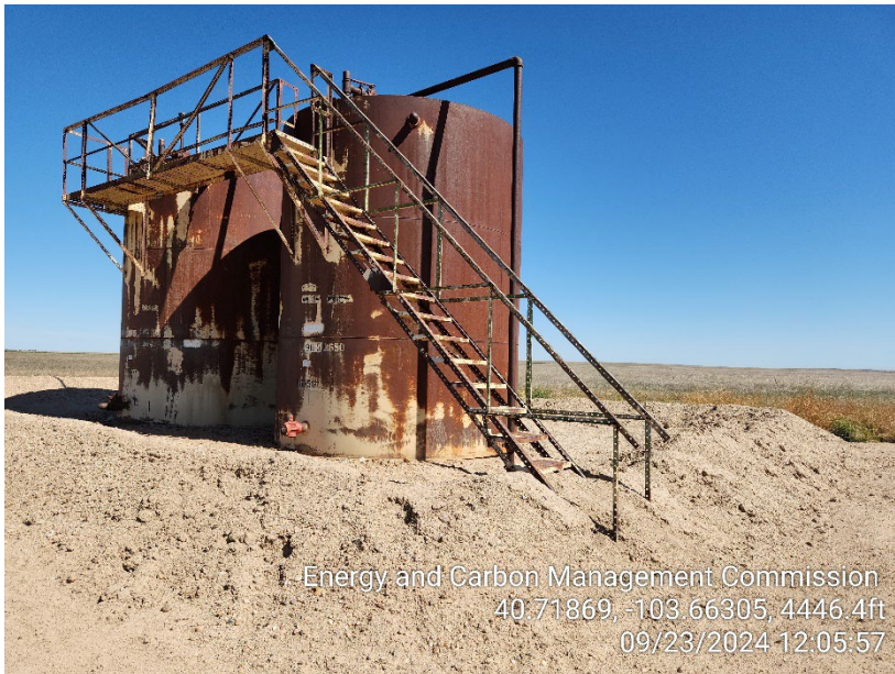
Photo 13 – Tank Battery – Berms Inadequate
