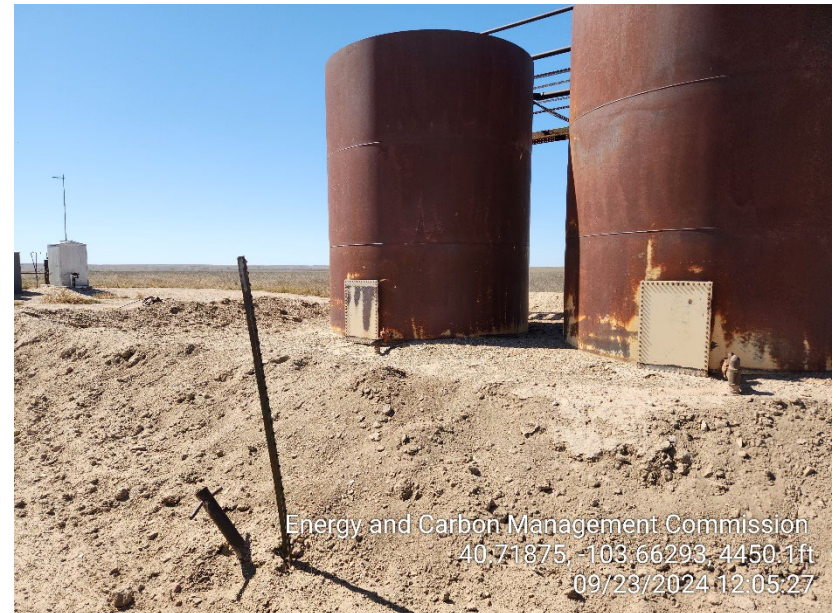
Photo 10 – Tank Battery – Berms Inadequate
