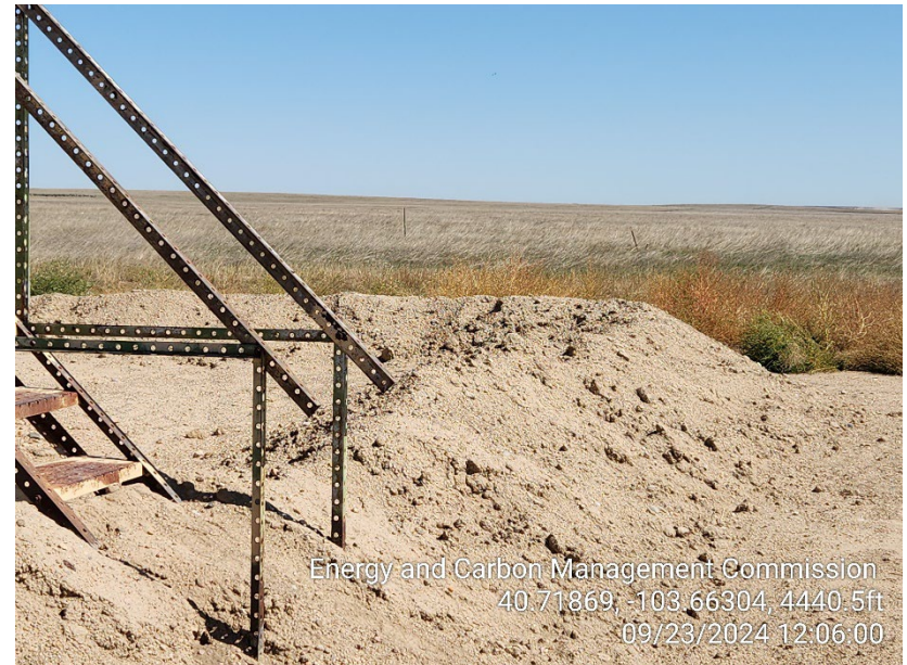
Photo 14 – Tank Battery – Berms Inadequate
