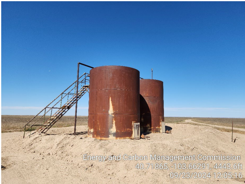
Photo 9 – Tank Battery – Berms Inadequate
