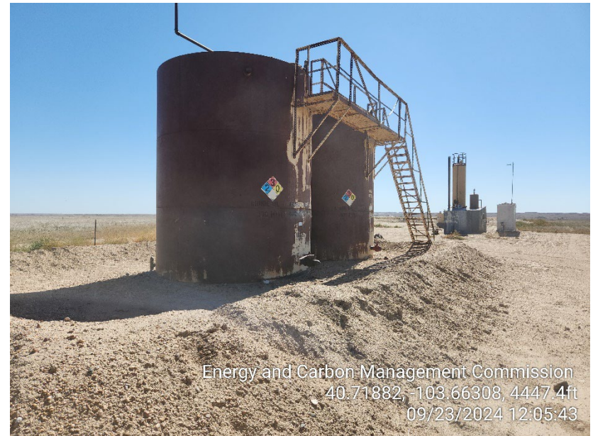
Photo 12 – Tank Battery – Berms Inadequate
