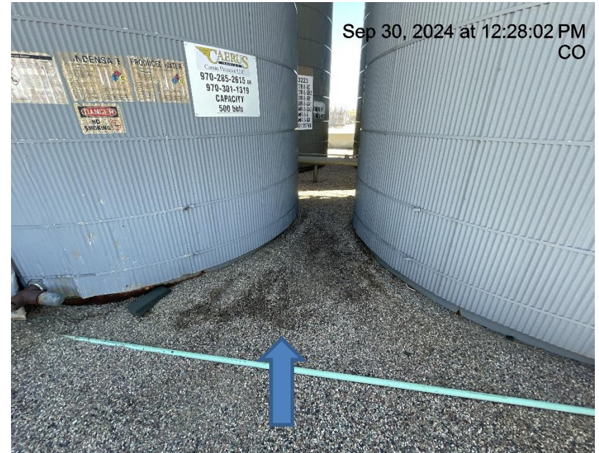
Photo # 2771 Staining in secondary containment
