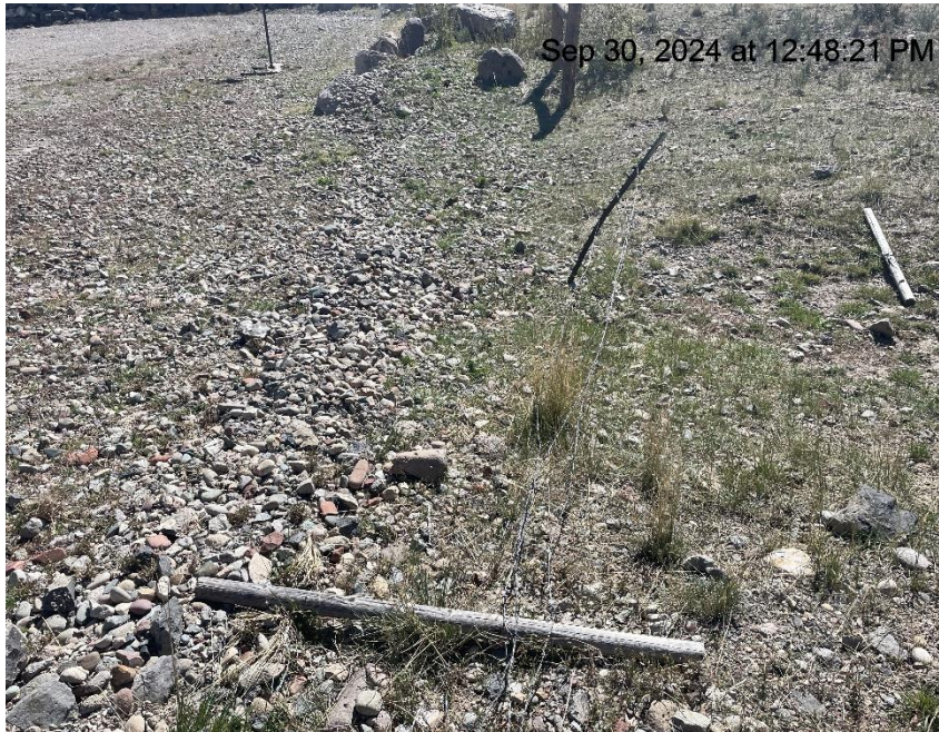
Photo # 2754 Barbed wire fence needs maintenance/wildlife hazard
