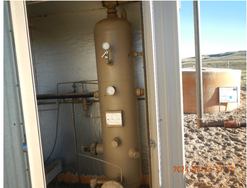
4. Vertical separator inside separator shed.
