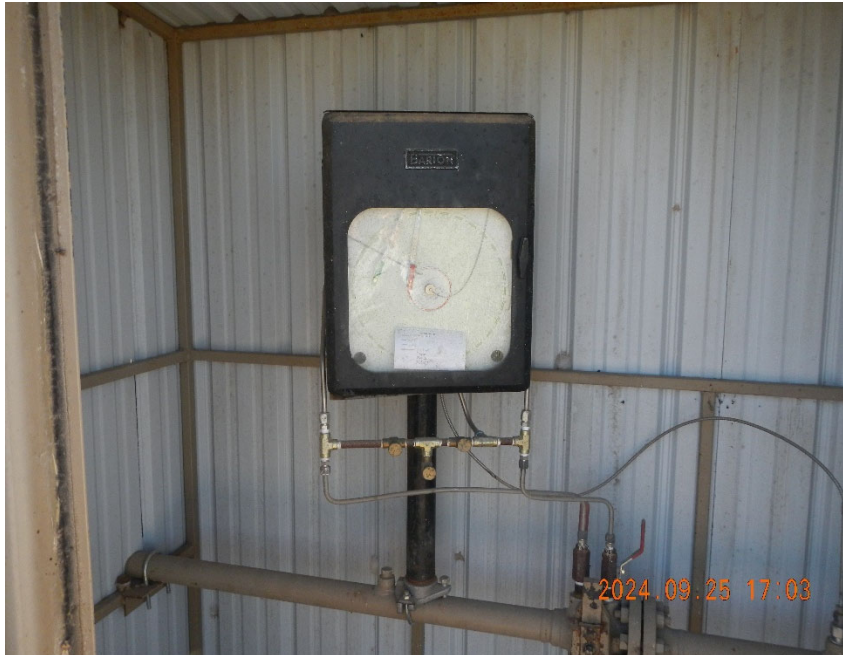
5. Gas meter inside meter shed.
