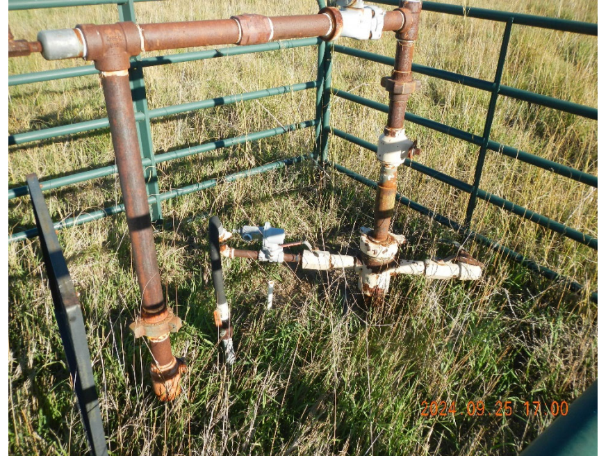
2. View of wellhead. Note vegetation inside fencing. Note white PVC pipe at center of frame.
