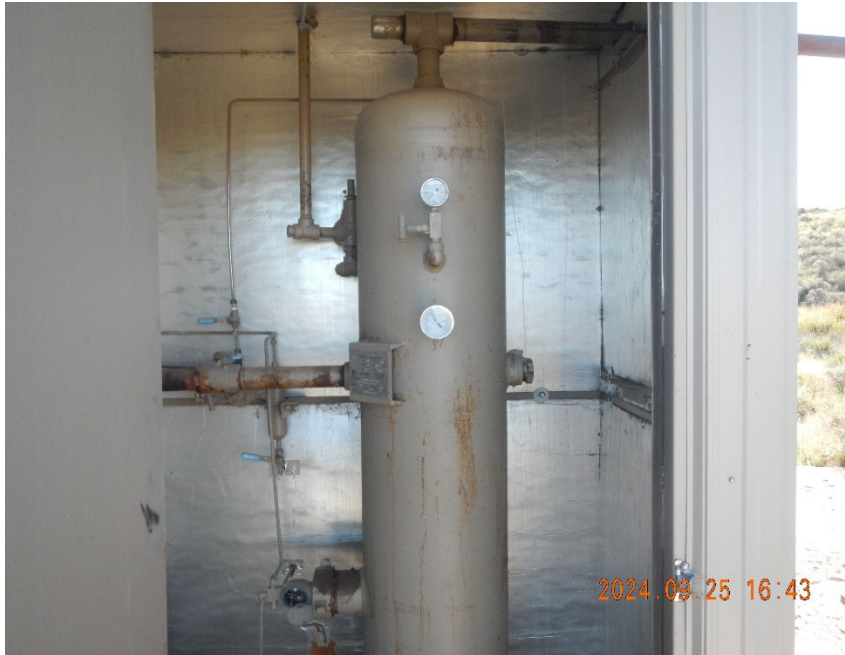
5. Vertical separator inside shed.
