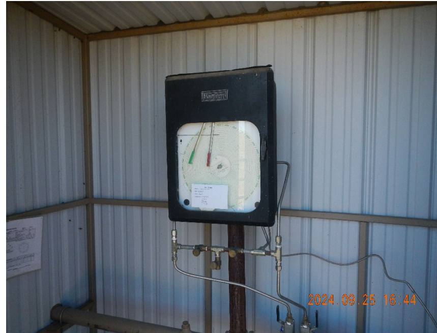
6. Gas meter inside meter shed.
