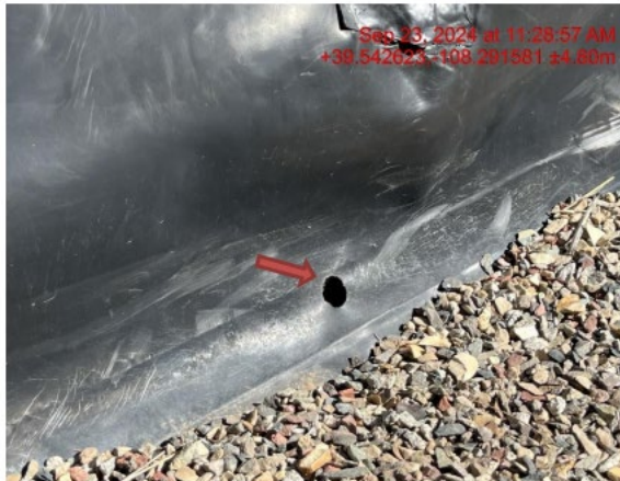
Hole in containment liner - Photo #06164
