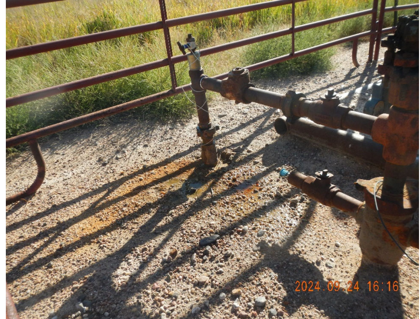
2. View of wellhead. Active release at check valve.
