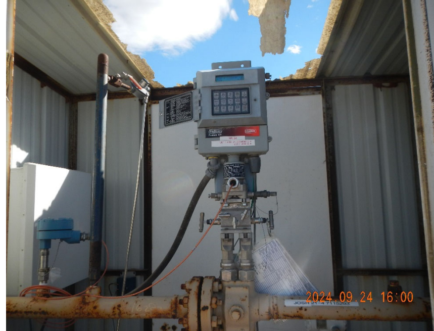
4. Gas meter inside shared meter shed.
