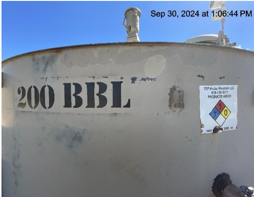
Photo # 2883 Tank labeled inaccurately/capacity incorrect
