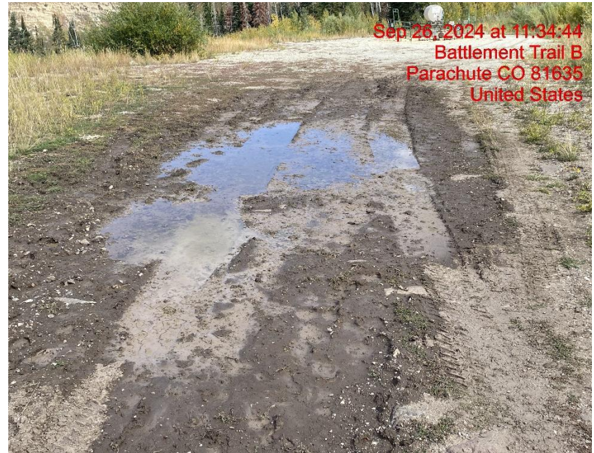
Lack of Stabilization with No Tracking BMP – Photo #03717
