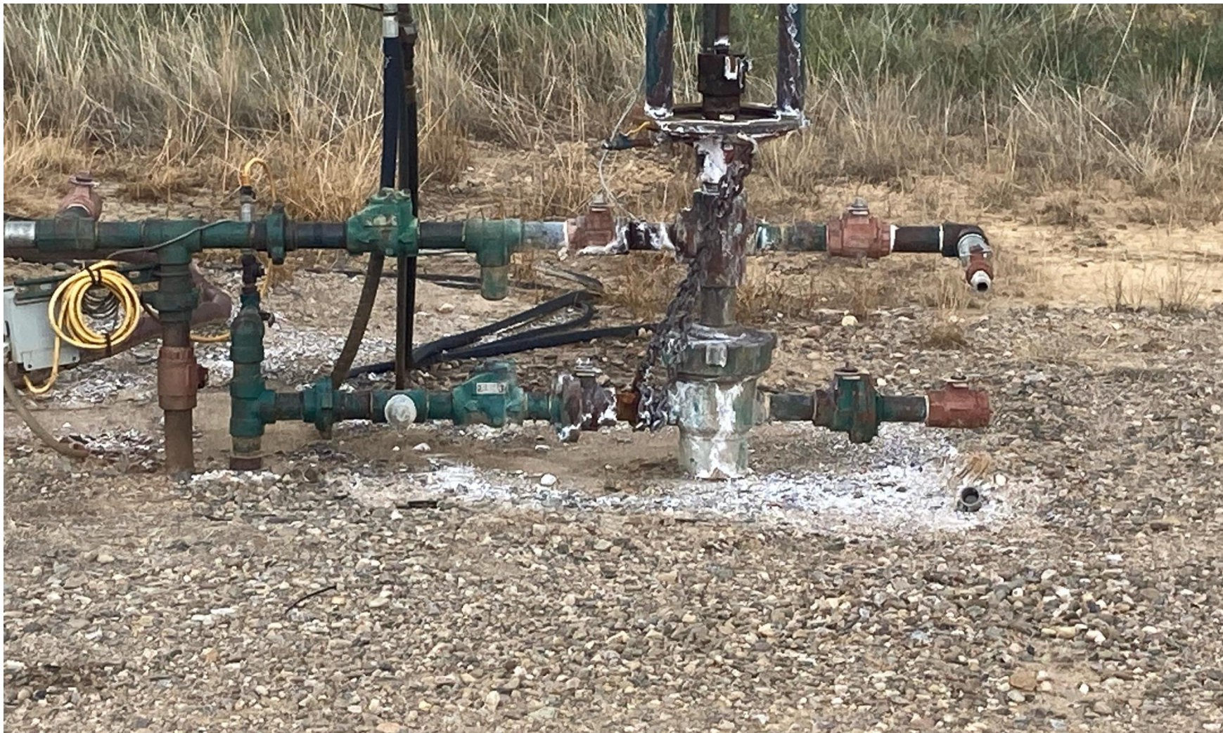
PHOTO 4: Produced water spill from the wellhead has left a salt impacted area around the wellhead. Securely fasten all valves, pipes, fittings, and Production Facilities to ensure good mechanical condition, inspect at regular intervals and maintain in good mechanical condition remove and dispose of impacted material per Rule 608.e. CA DATE 10/30/2024.
