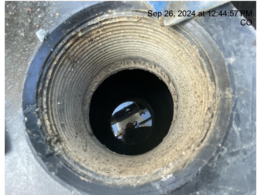
Photo # 2139 Failure to maintain chemical BMP/chemical tank containment approximately 3/4 th full of fluid/BMP insufficient to contain possible spill
