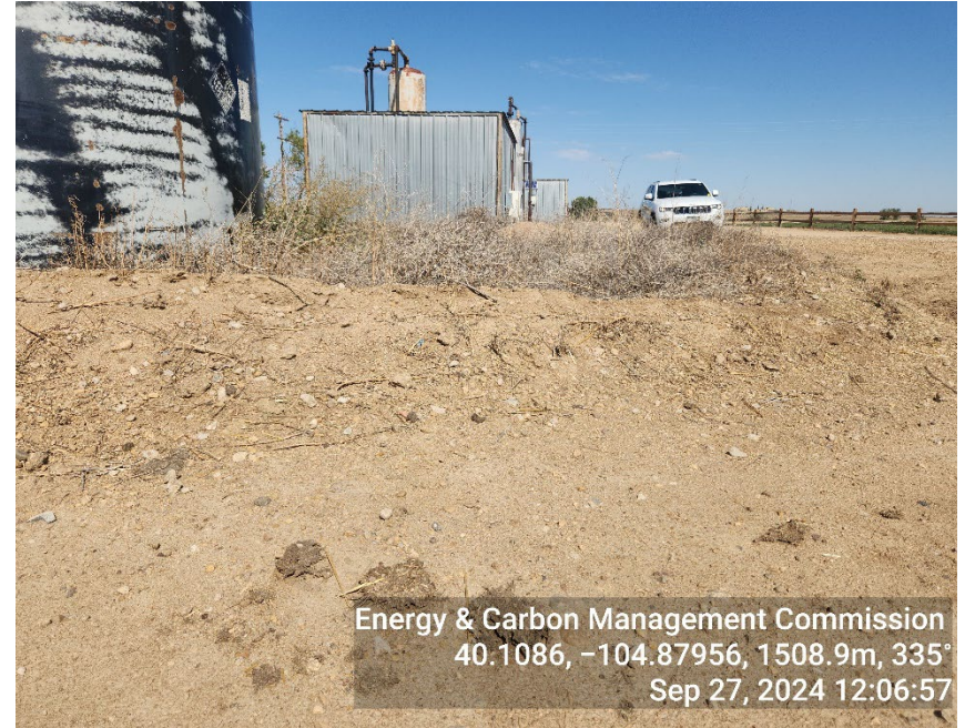
Photo 2: Berm not maintained, overgrown vegetation
