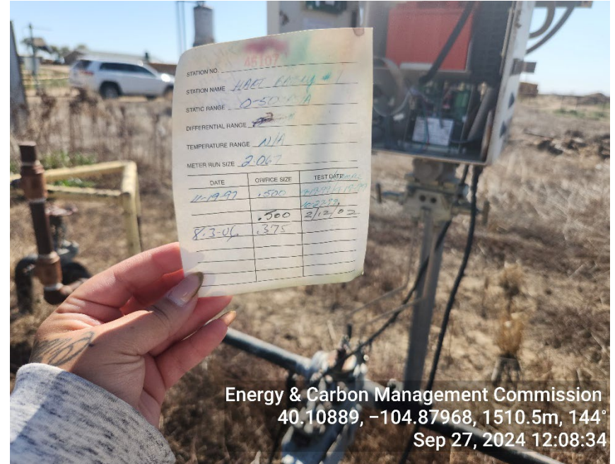
Photo 6: Meter not annually calibrated.
