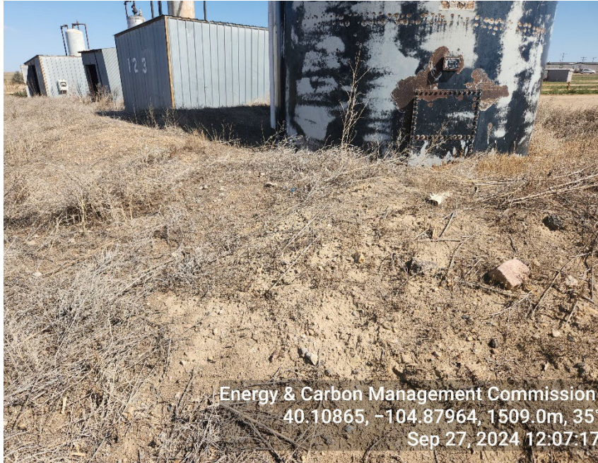
Photo 5: Berm not maintained, overgrown vegetation
