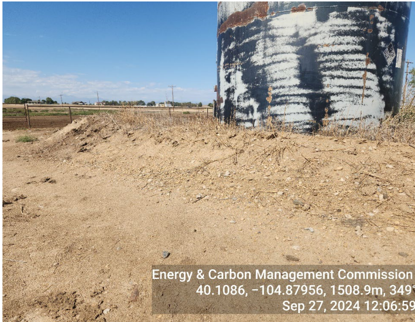
Photo 3: Berm not maintained, no sign on tank
