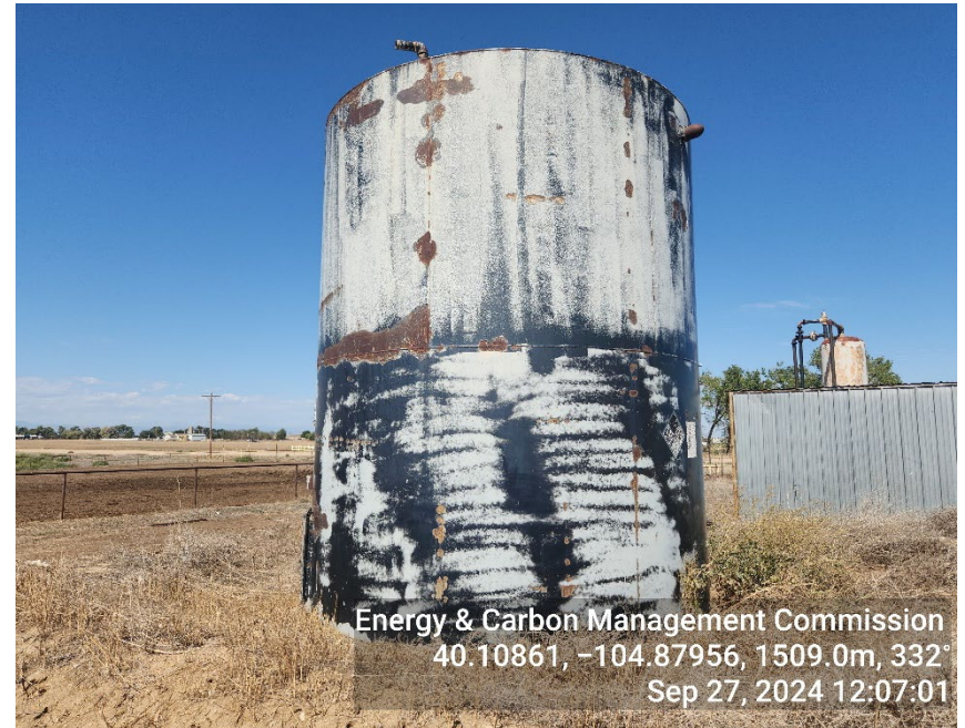
Photo 4: No sign on tank (capacity/contents/NFPA)
