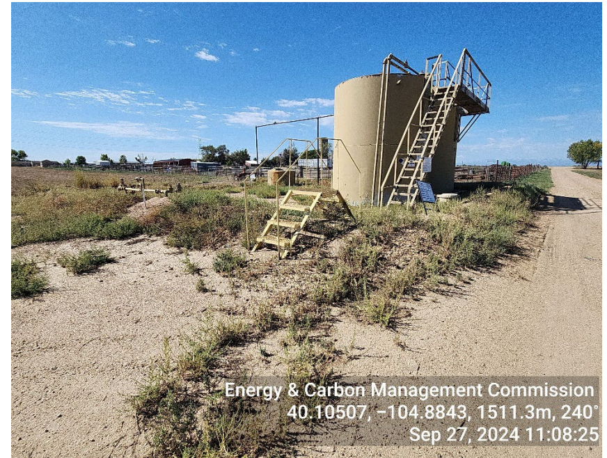
Photo 10: Overgrown vegetation, berm not well maintained
