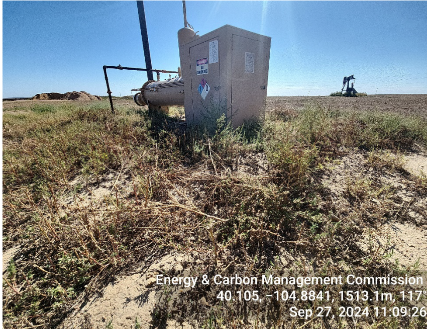
Photo 13: Overgrown vegetation, berm not well maintained
