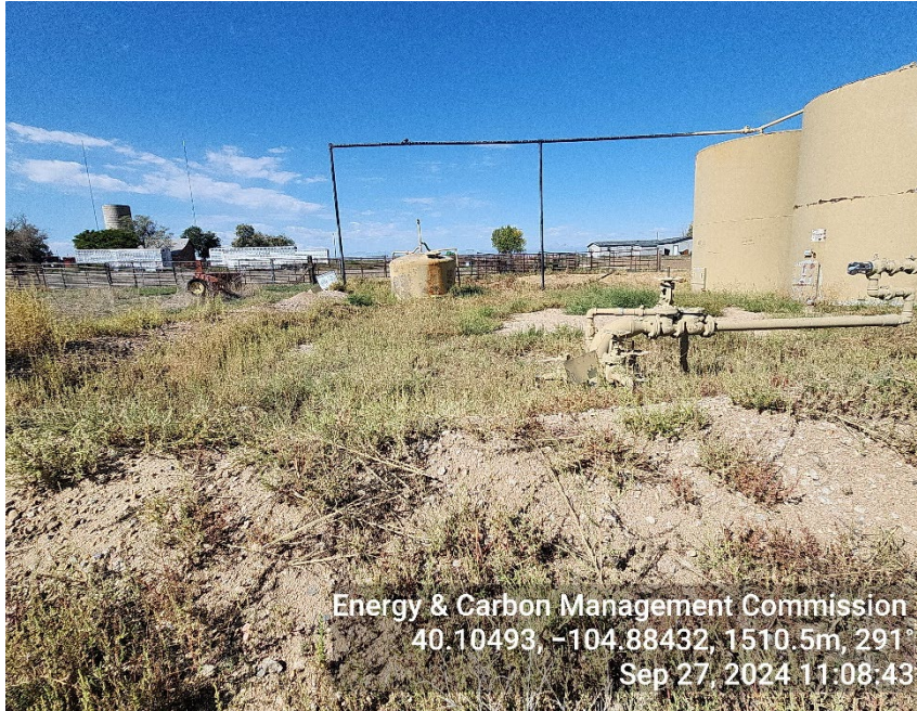
Photo 11: Overgrown vegetation, berm not well maintained
