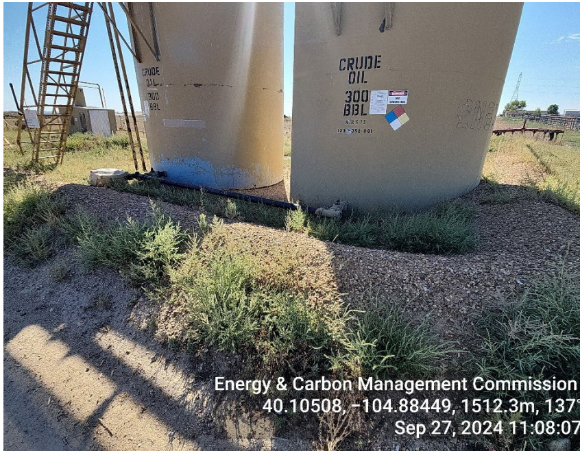
Photo 9: Overgrown vegetation, berm not maintained
