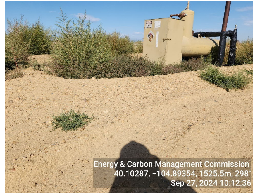
Photo 10: Earthen berm not maintained
