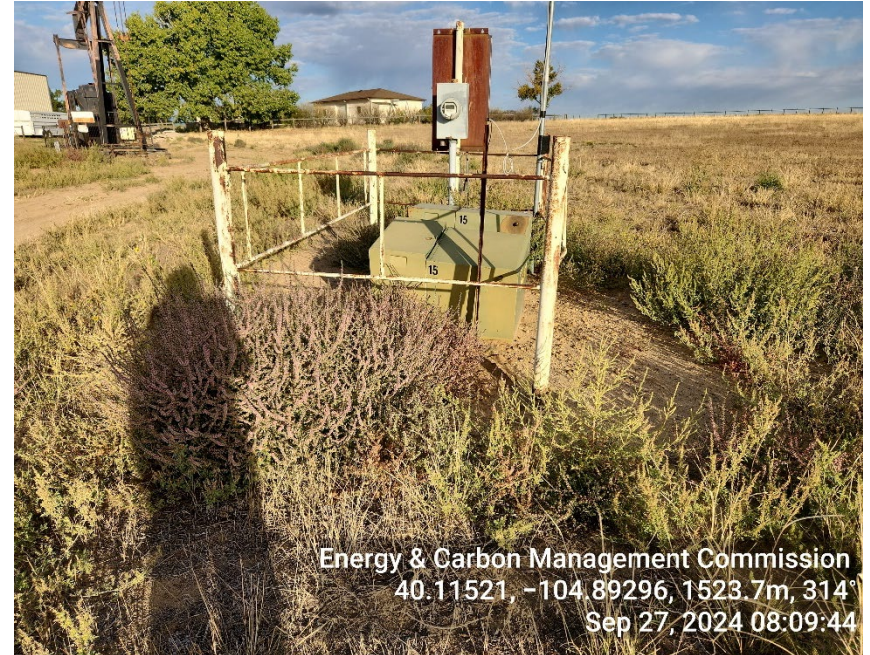
Photo 2: Overgrown vegetation around ancillary equipment
