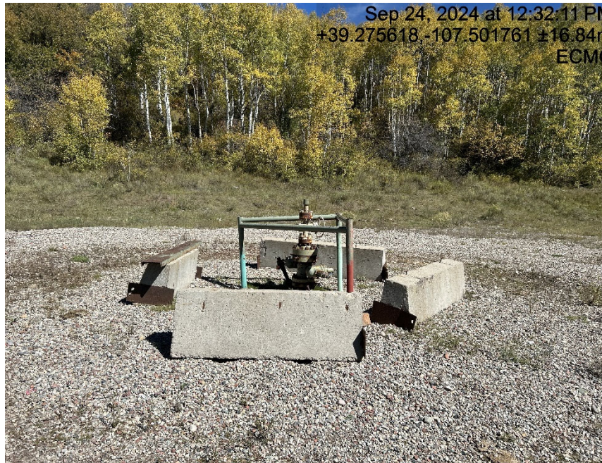
Well head lacking signage
