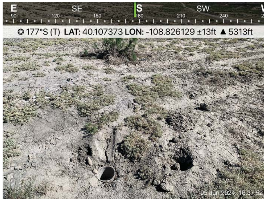
Photo 4: Silver King Pan Am Hayes #5-27 (OWP) P&A wellhead, no methane detected, view south.
