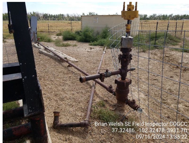
4. Wellhead with water leg disconnected
