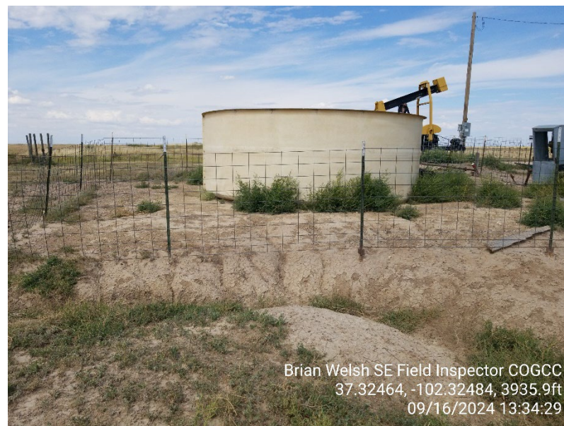
2. Erosion on south side of location around water tank
