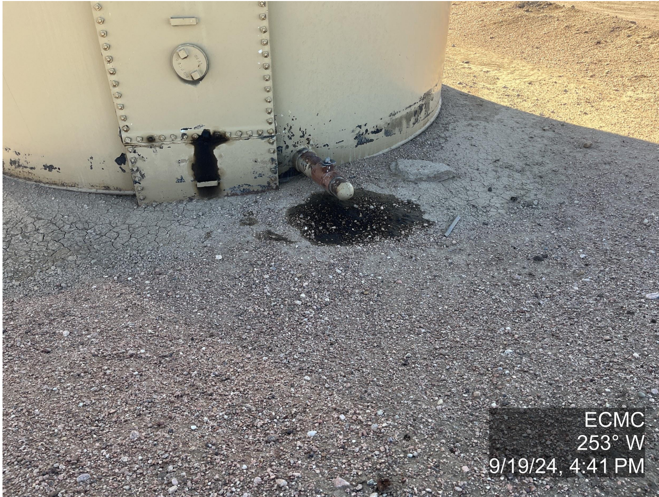
Photo 9. The photo was taken at the tank battery location facing West. The photo illustrates stained soil within secondary containment at the tanks.
