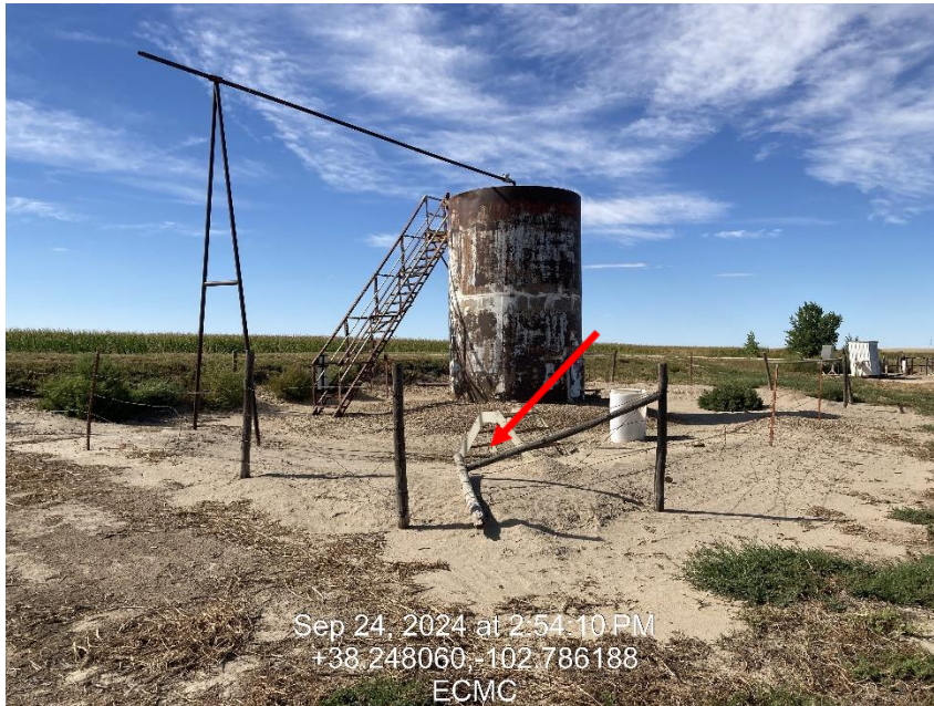
Photo 7 – Tank Battery fencing in disrepair
