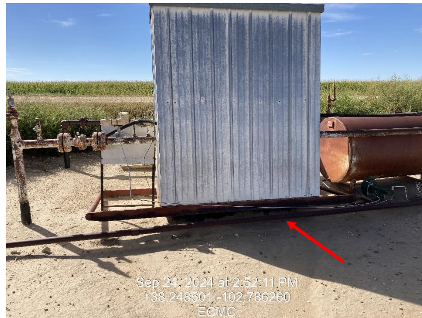
Photo 4 – Meter house settling
