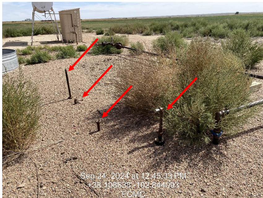
Photo 5 – Pipe risers not capped and no OOSLAT
