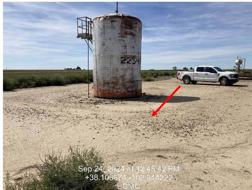
Photo 6 – Tank Battery, Secondary Containment not adequate
