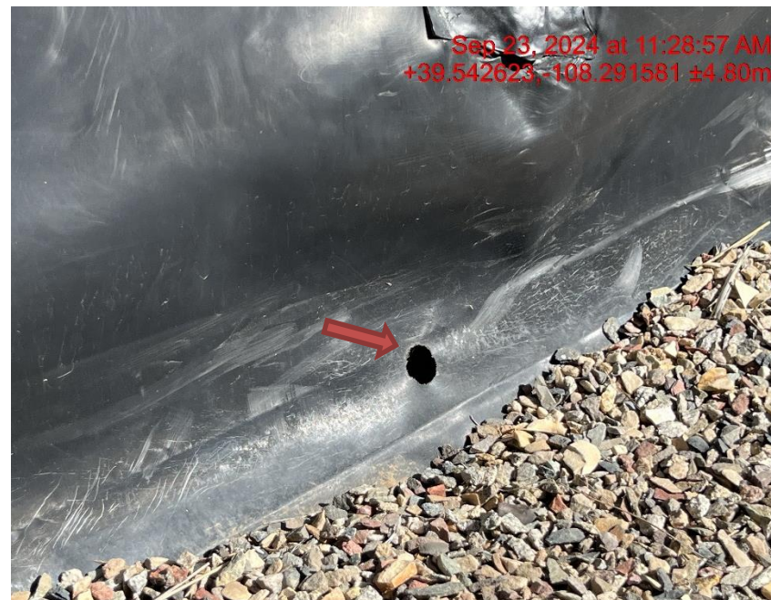
Hole in containment liner - Photo #06164
