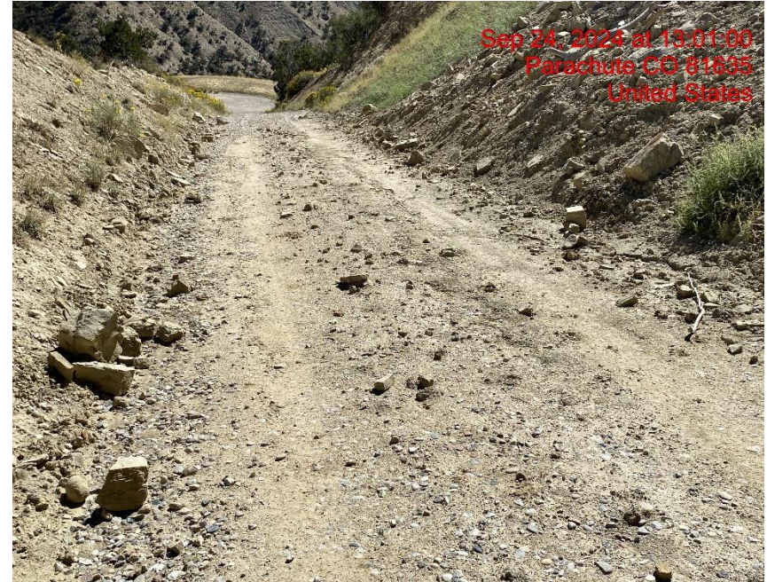
Cut Slope Eroding onto Access Road – Photo #03649
