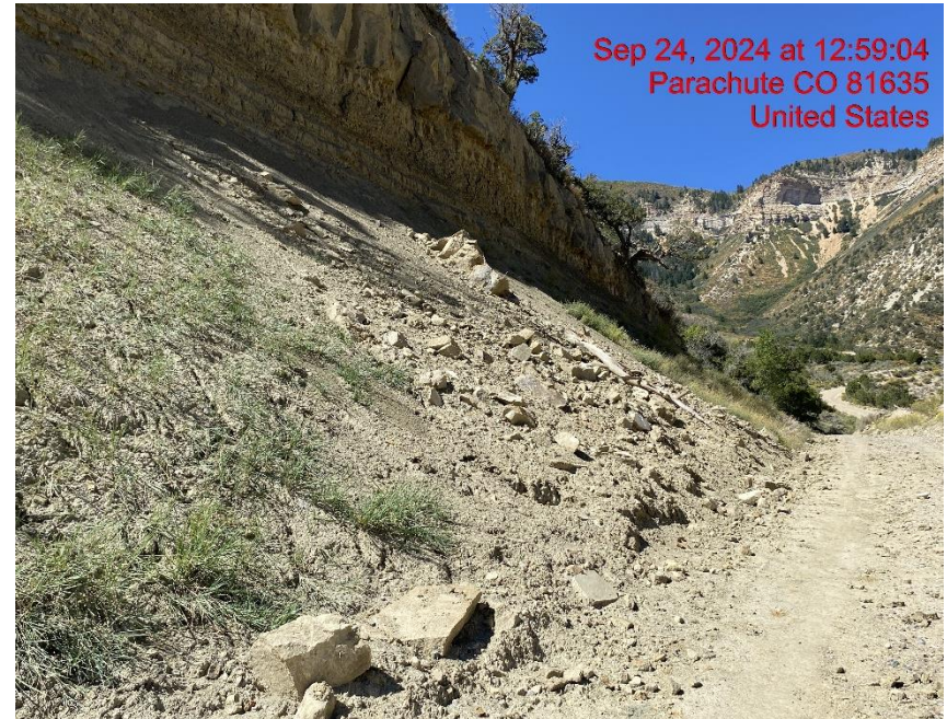
Unstabilized Cut Slope – Photo #03647
