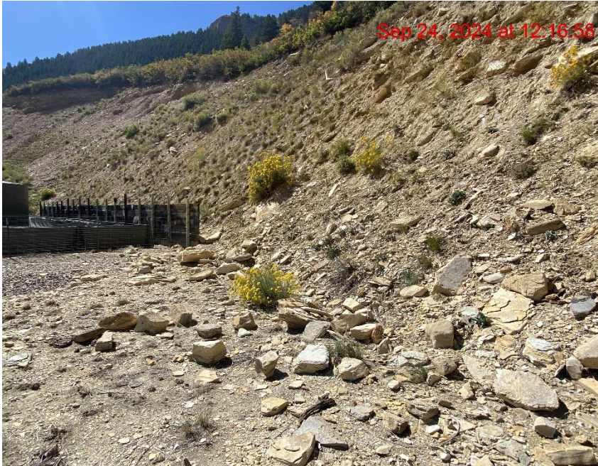
Unstabilized Cut Slope – Photo #03604
