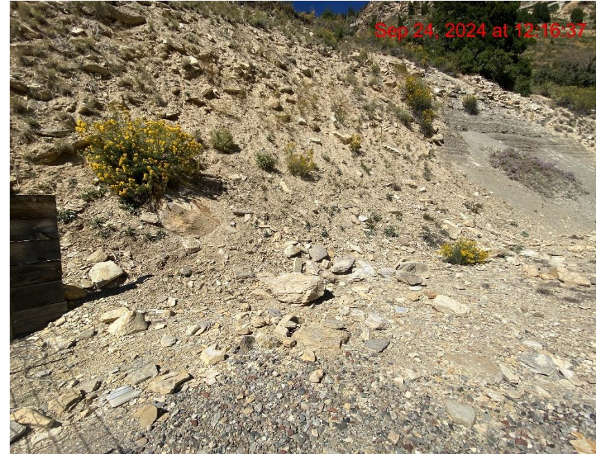
Unstabilized Cut Slope – Photo #03603
