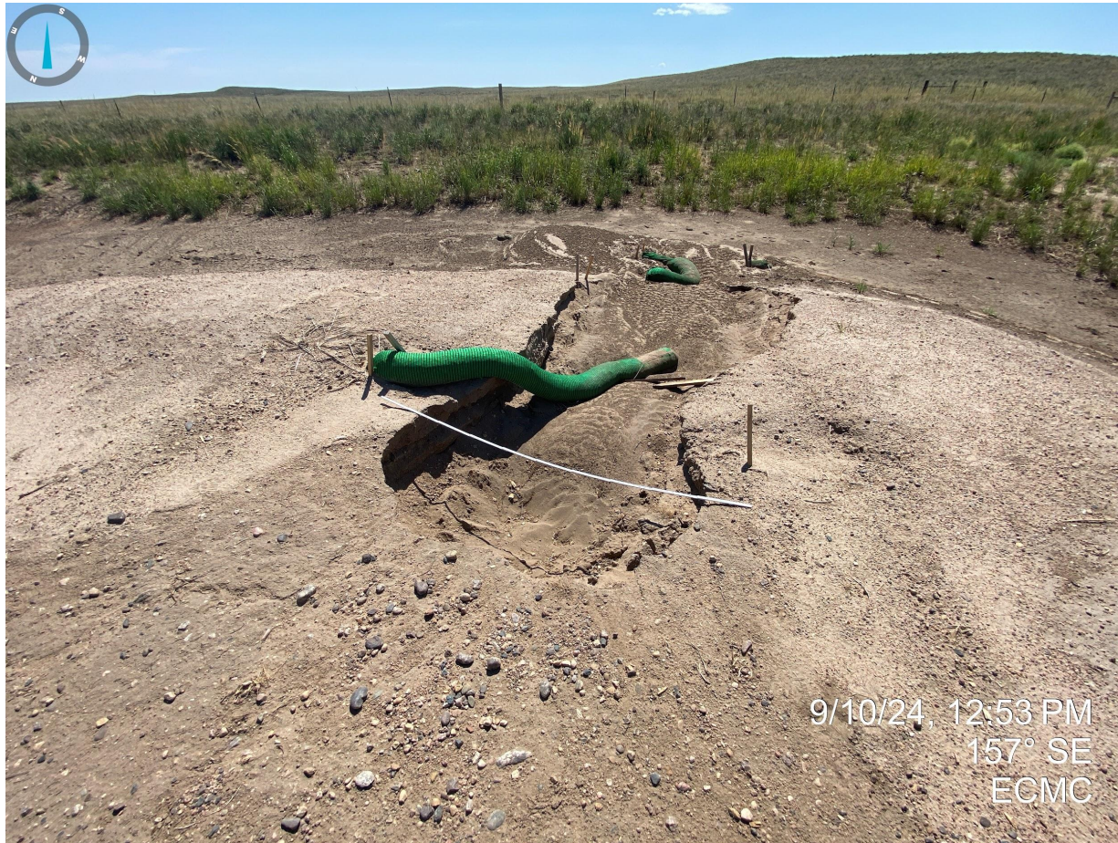
Photo 21. Erosion degradation near the southwest corner of the drilling pad, near the sediment detention area.
