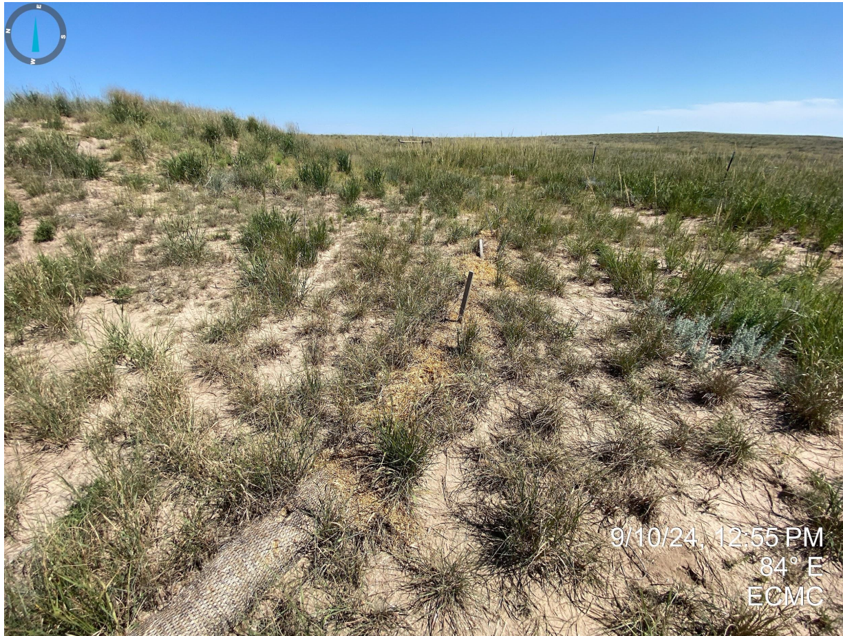
Photo 25. Degraded straw wattles around the topsoil stockpile need to be removed as it's considered debris.
