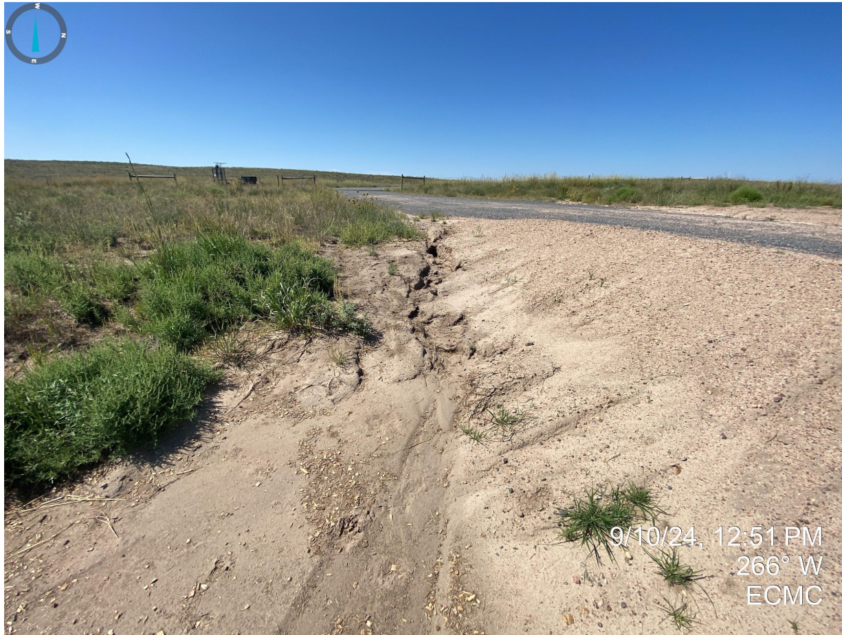
Photo 20. Erosion degradation observed near the entrance to the drilling pad.
