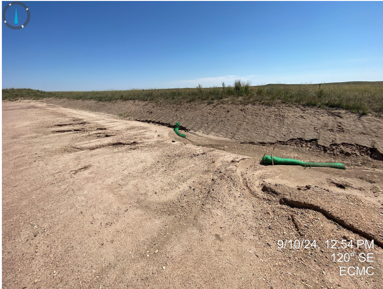
Photo 22. Erosion degradation observed on the southern portion of the drilling pad.
