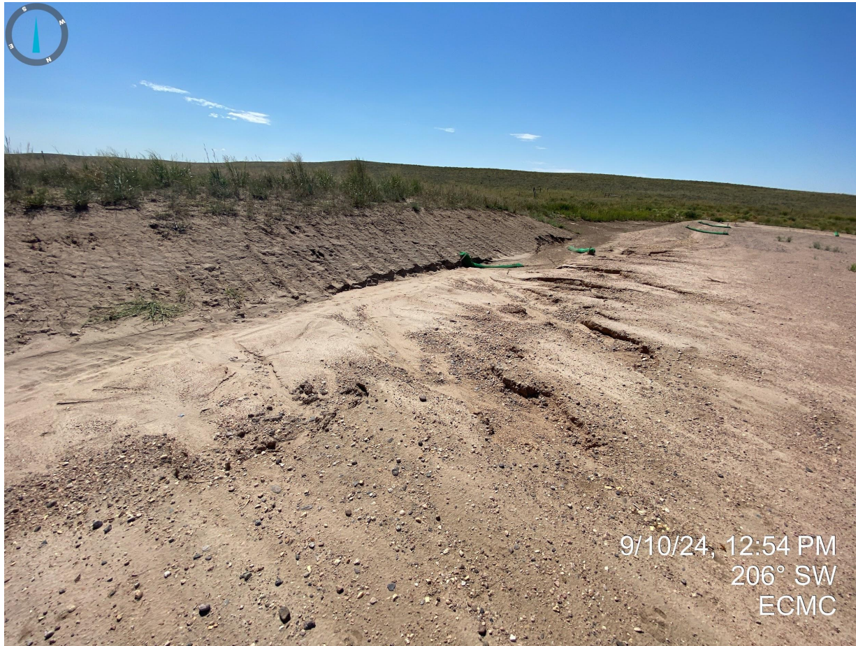
Photo 23. Erosion degradation observed on the southern portion of the drilling pad.
