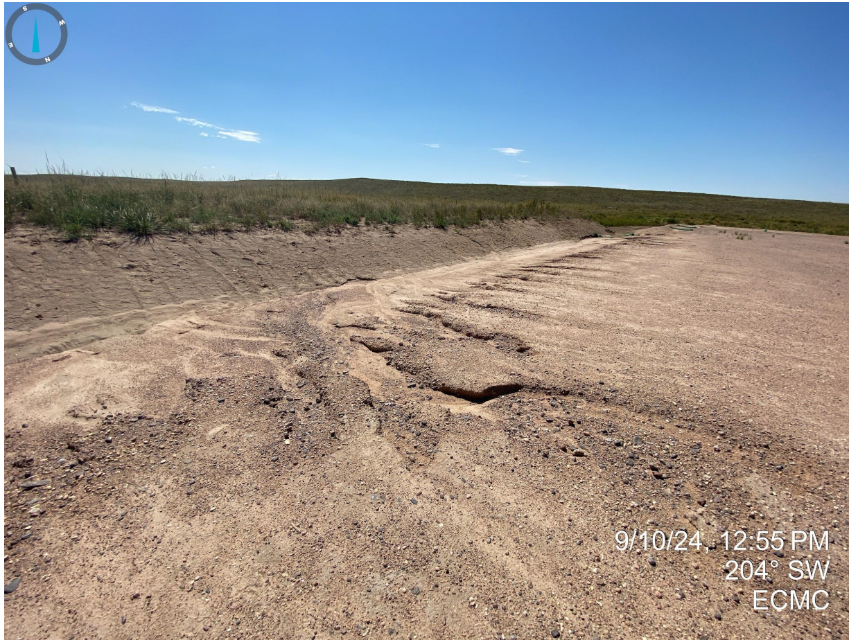
Photo 24. Erosion degradation observed on the southern portion of the drilling pad.
