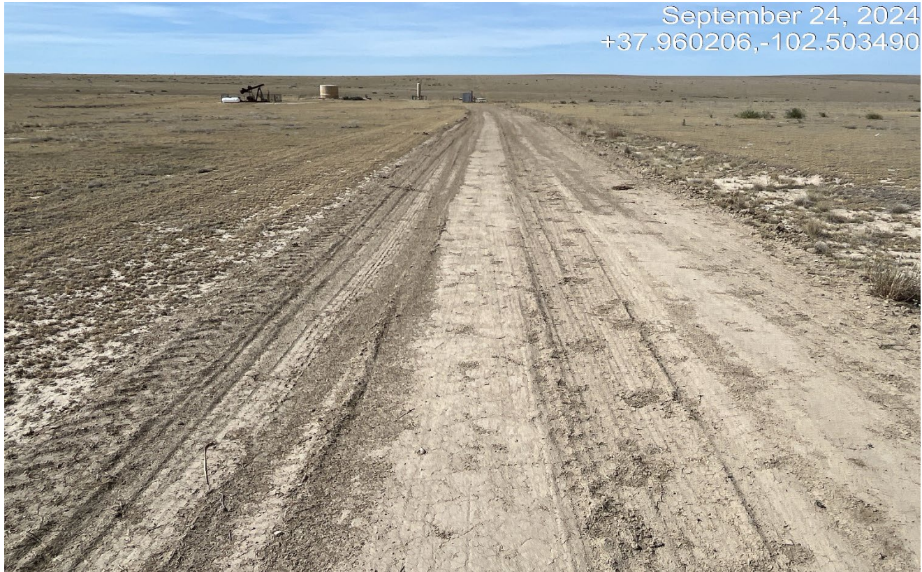
Photo 1. Facing east along the access road. The ruts along the road have been repaired but no stabilization was performed to prevent erosion reoccurrence.
