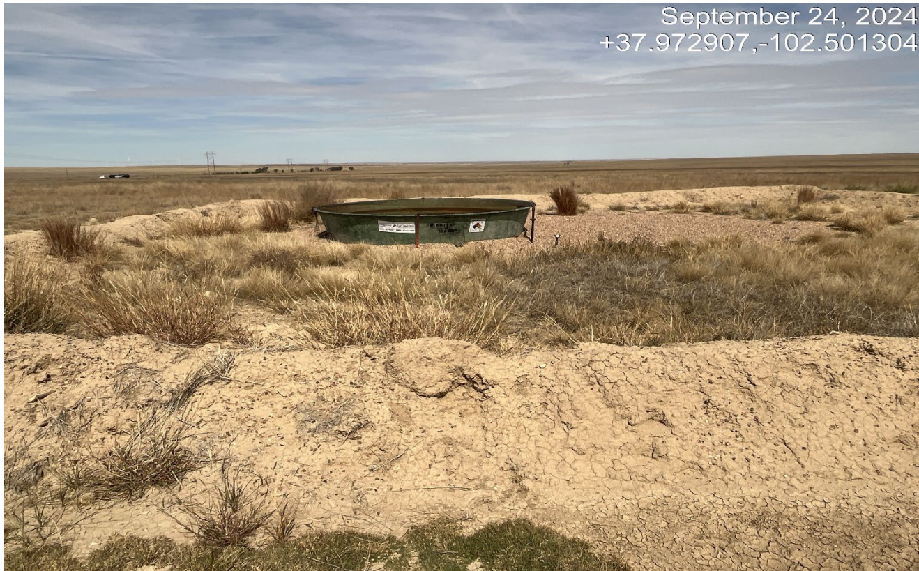
Photo 2. The berm has been built up better for secondary containment and netting has been placed over the tank. Labels are posted on the tank.
