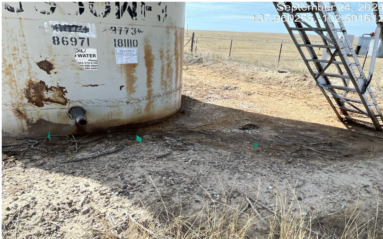
Photo 4. There is stained soils still observed inside the secondary from the previous spill. There are green flags put around the impacted area.
