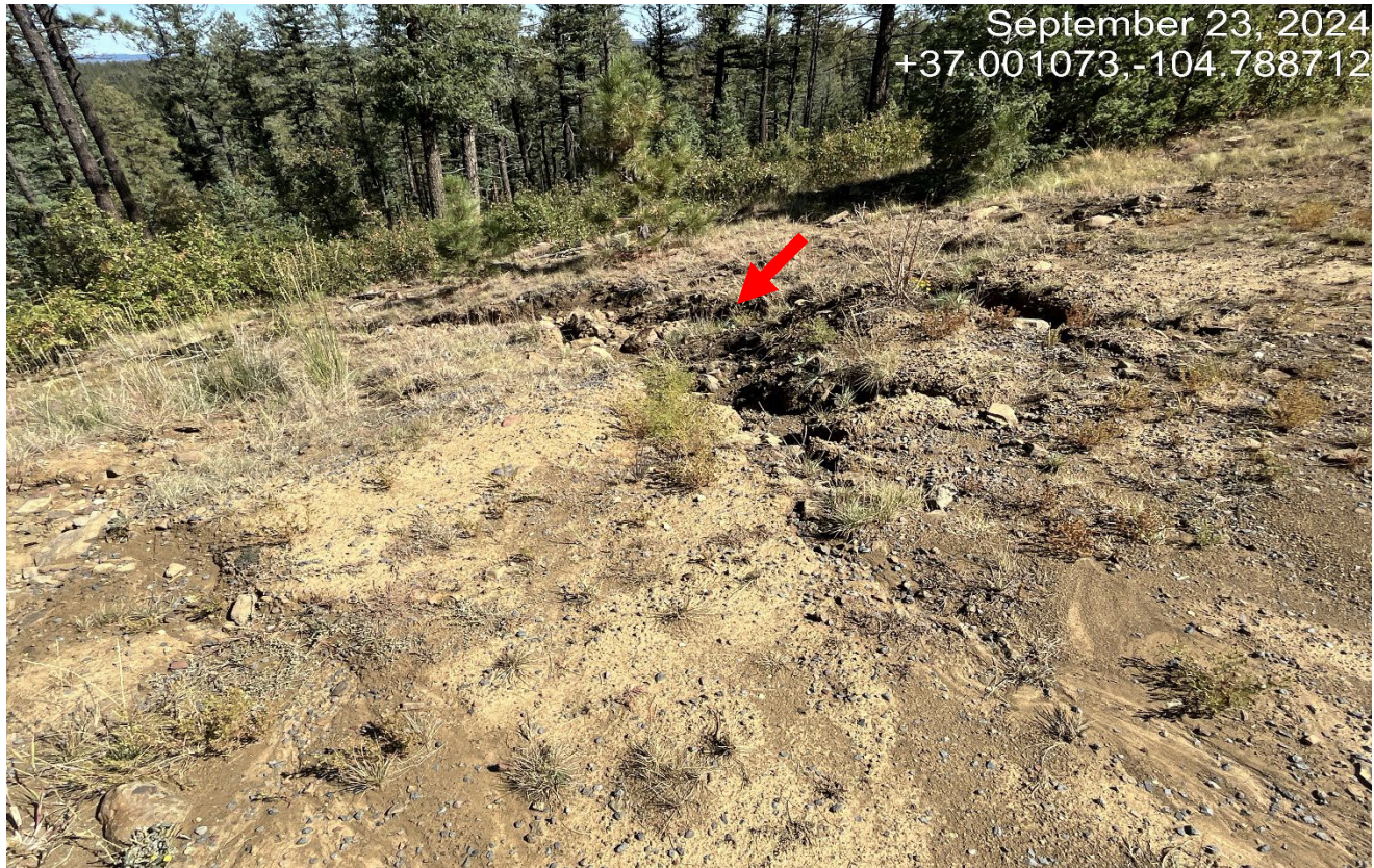
Photo 4. There is an erosion channel at the northeast side of the location that needs to be repaired. Previous CA was not completed.
