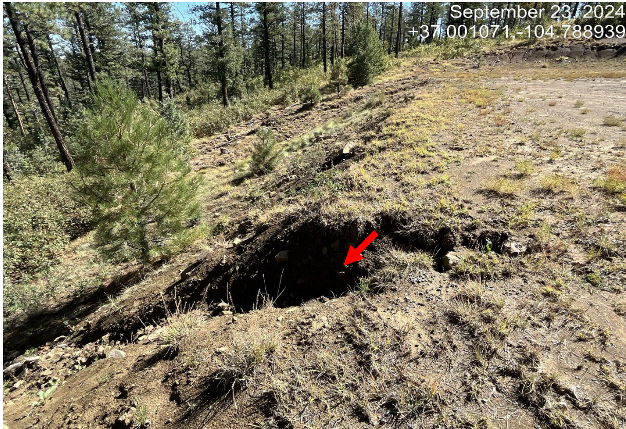
Photo 3. There are other erosion channels along the cut slope that have not been repaired.
