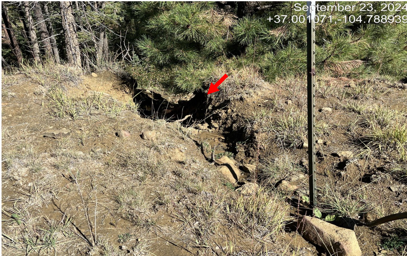
Photo 2. There is an erosion channel at the northwest side of the location that needs to be repaired. Previous CA was not completed.
