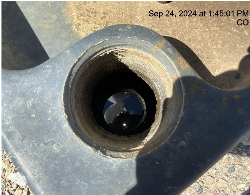
Photo # 1702 Failure to maintain chemical BMP/chemical tank containment approximately 3/4 th full of fluid/BMP insufficient to contain possible spill
