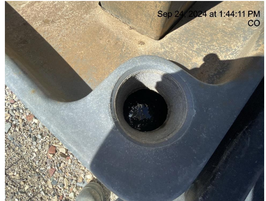
Photo # 1703 Failure to maintain chemical BMP/chemical tank containment approximately 3/4 th full of fluid/BMP insufficient to contain possible spill
