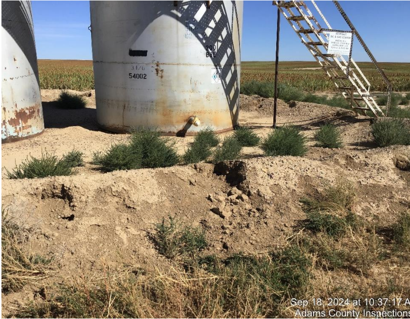
Photo #3 Damaged berm and weeds in and on berm.
