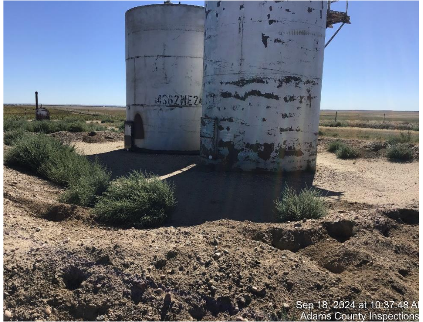
Photo #4 Damaged berm and weeds in berm.
