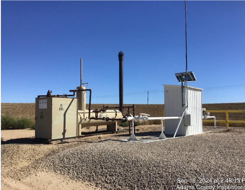
Photo #3 Separator and Meter house.
