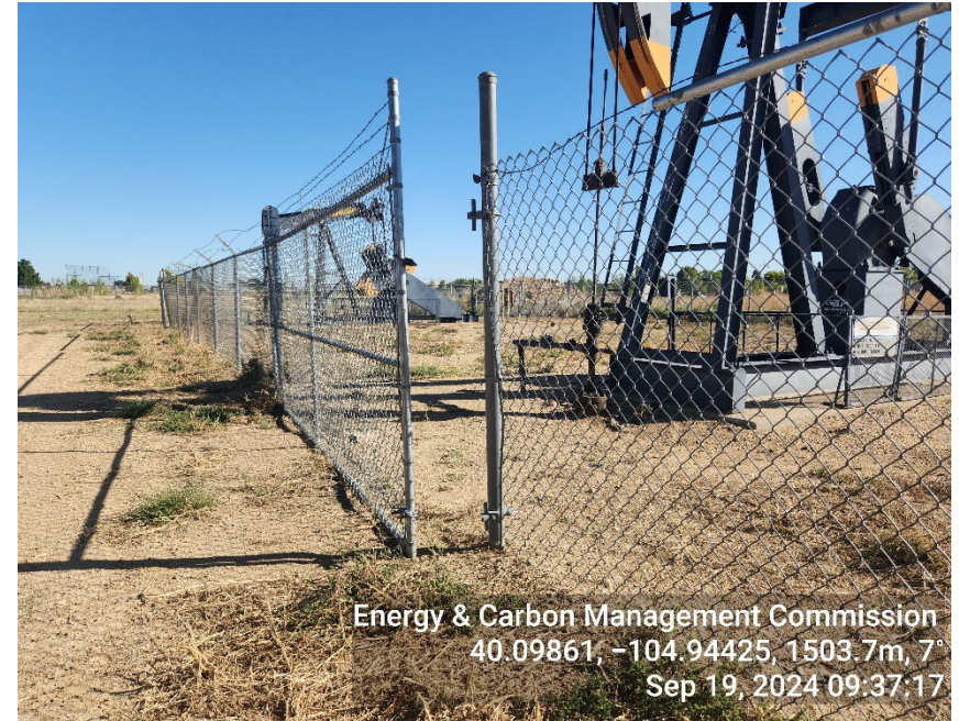
Photo 18: Fencing in disrepair
