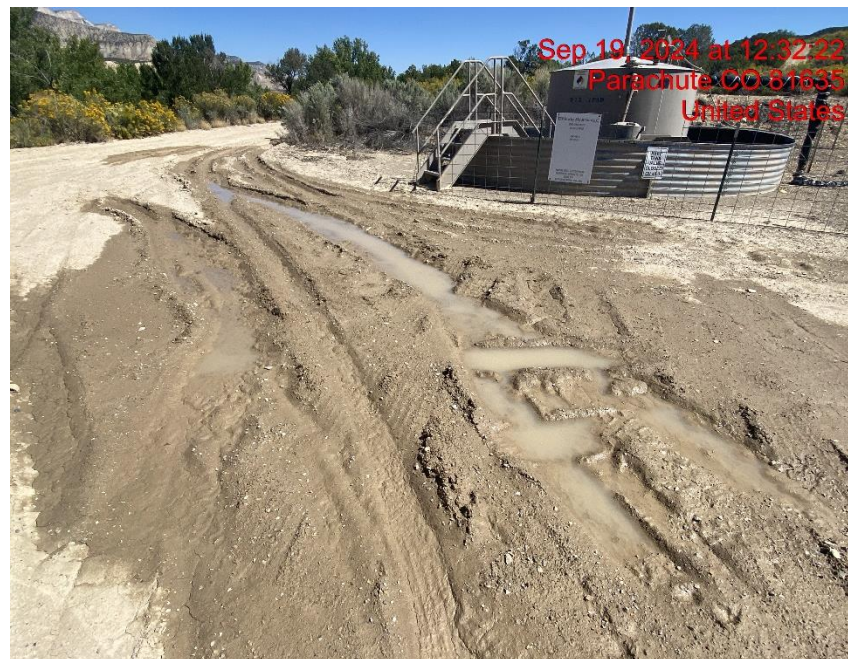
Lack of Stabilization – Photo #03545
