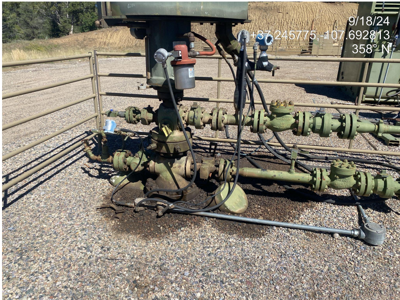
Photo 3. View of impacted surface material observed at the well head.
