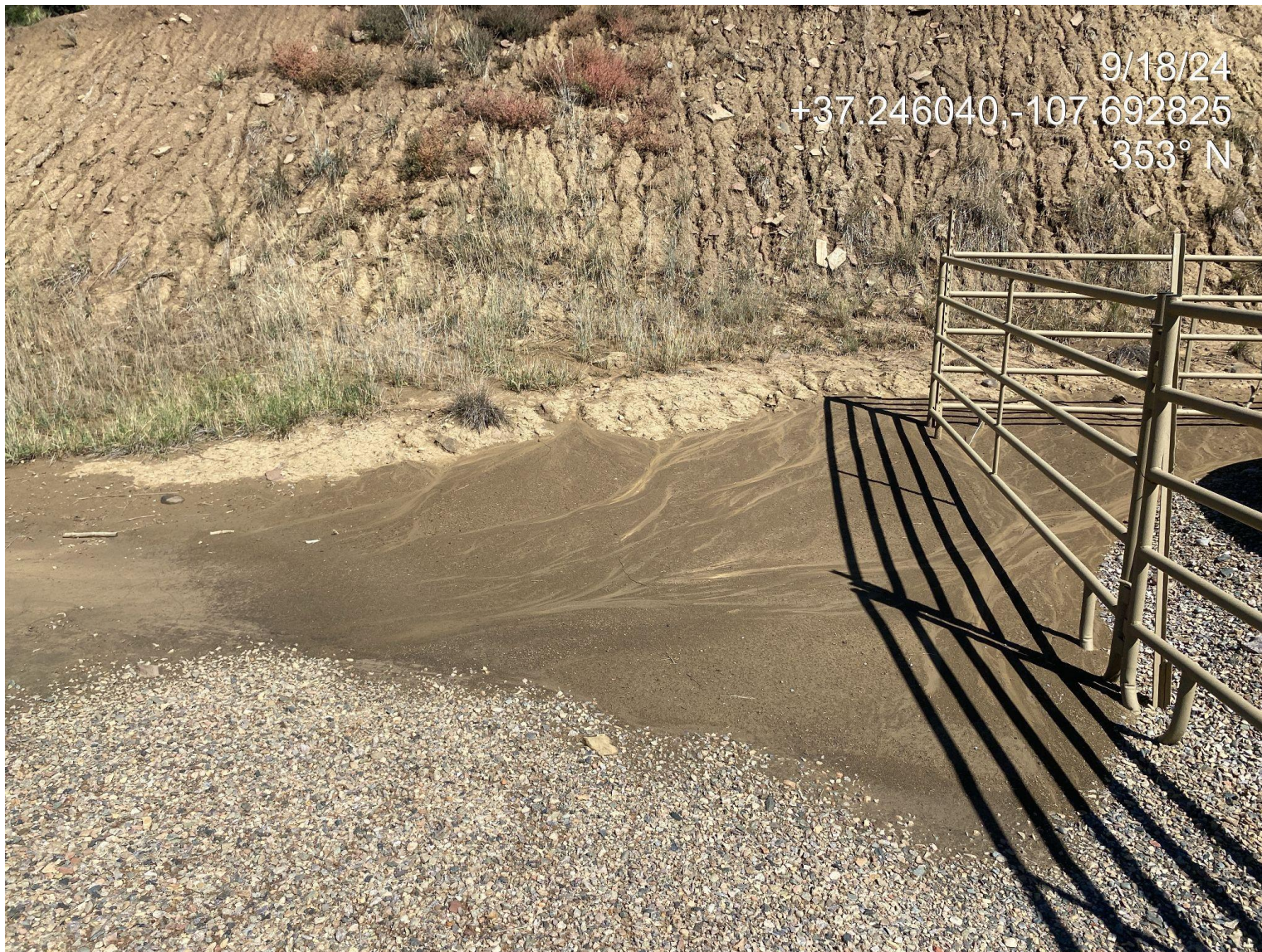
Photo 5. Evidence of sediment transport/deposition coming off the bare cutslope.
