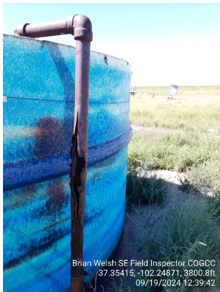
3. Water leg corrosion
