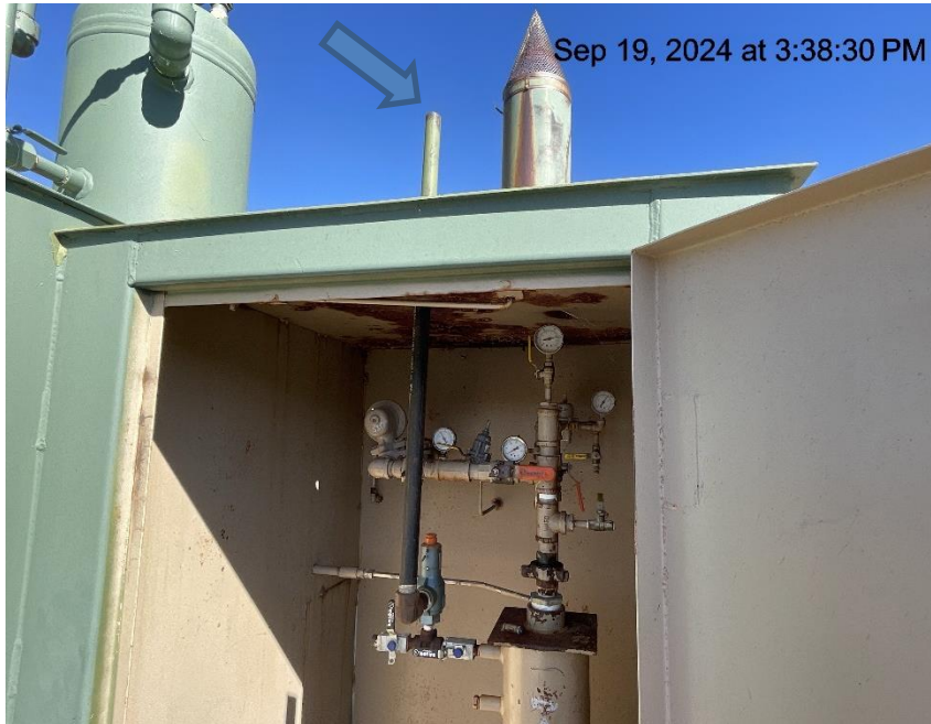
Photo # 1245 PRV vent line does not comply with CECMC pressure safety device rules
