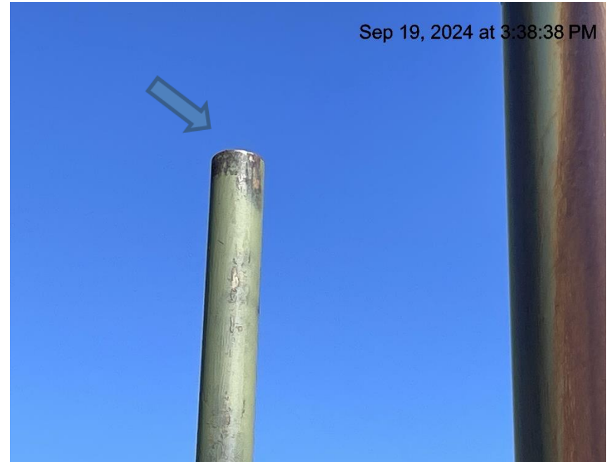
Photo # 1246 PRV vent line does not comply with CECMC pressure safety device rules
