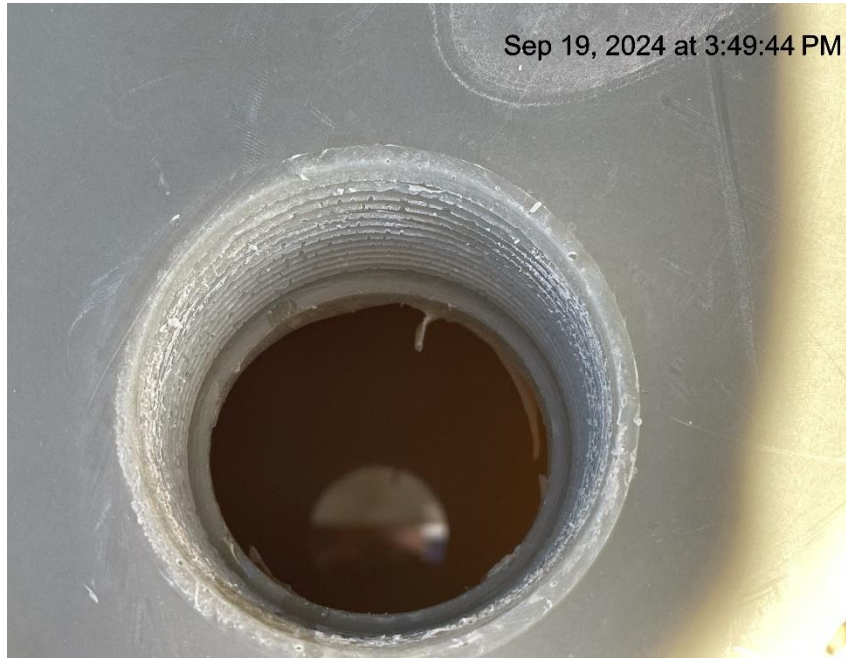
Photo # 1247 Failure to maintain chemical BMP/chemical tank containment approximately 3/4 th full of fluid/BMP insufficient to contain possible spill
