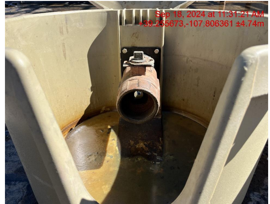
Open ended load line - Photo #05955
