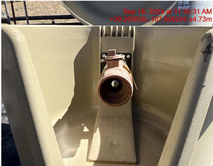
Open ended load line - Photo #05954
