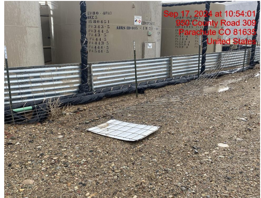
Damaged Battery Fencing – Photo #03457
