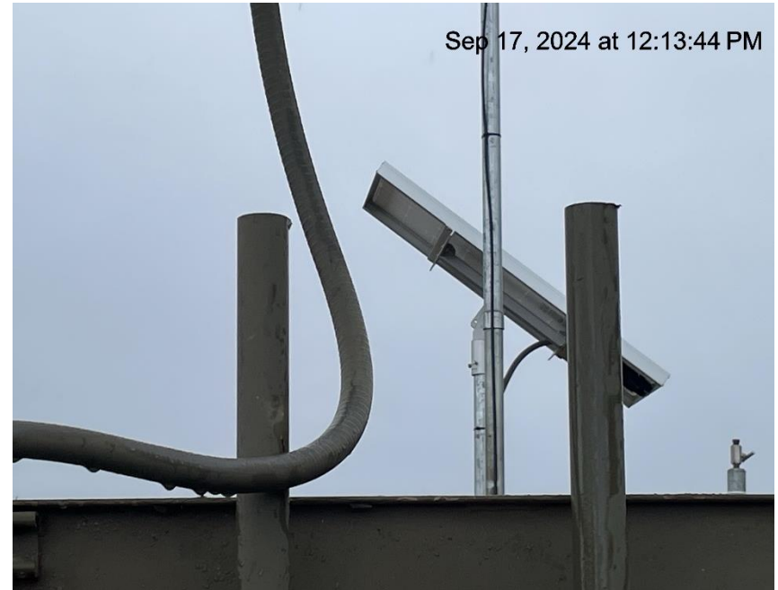
Photo # 667 PRV & rupture disc vent lines do not comply with CECMC pressure safety device rules
