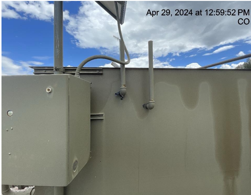
Photo # 5373 From inspection 708903672 conducted on 04/29/2024 PRV & rupture disc vent lines do not comply with CECMC pressure safety device rules
