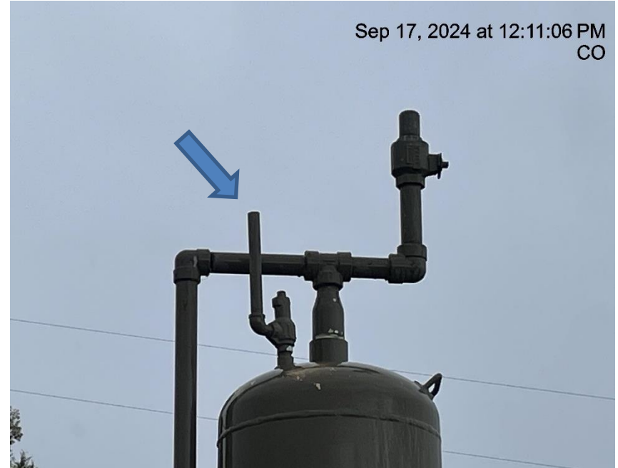
Photo # 668 PRV vent line does not comply with CECMC pressure safety device rules
