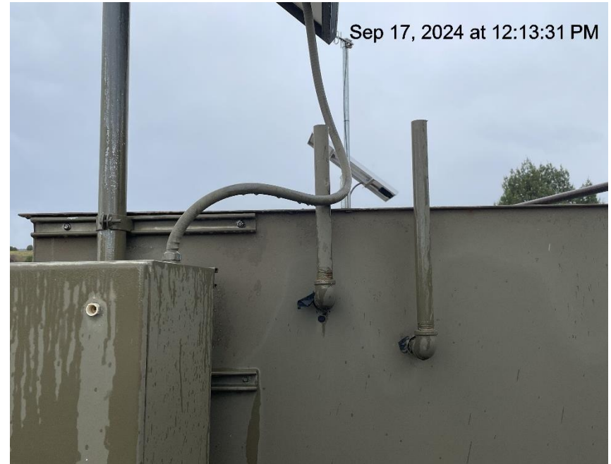
Photo # 666 PRV & rupture disc vent lines do not comply with CECMC pressure safety device rules
