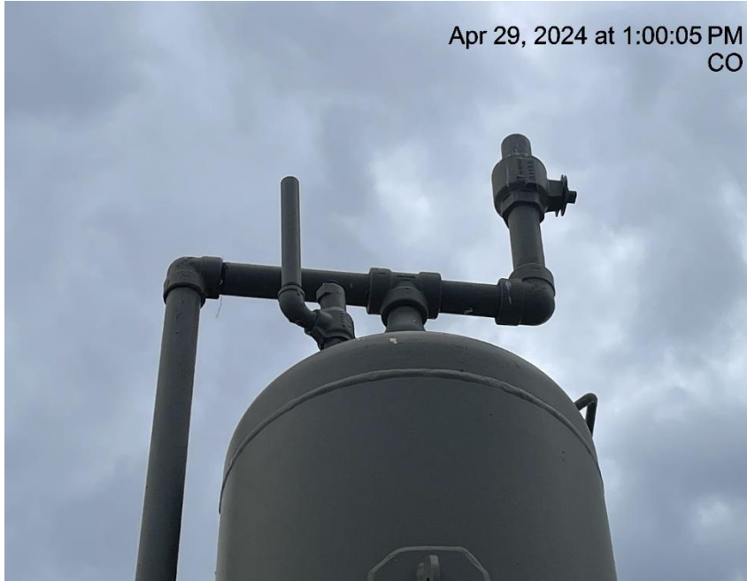
Photo # 5375 From inspection 708903672 conducted on 04/29/2024 PRV vent line does not comply with CECMC pressure safety device rules
