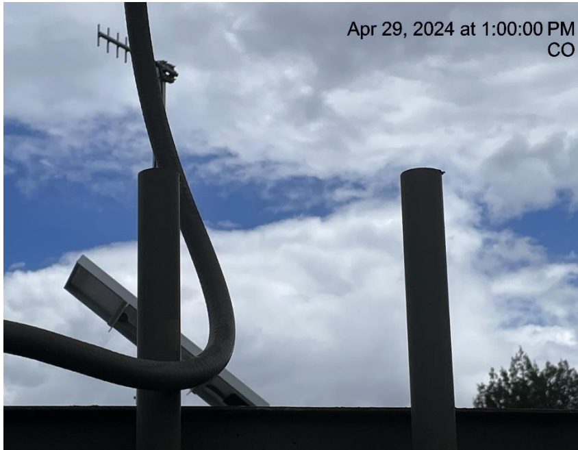
Photo # 5374 From inspection 708903672 conducted on 04/29/2024 PRV & rupture disc vent lines do not comply with CECMC pressure safety device rules
