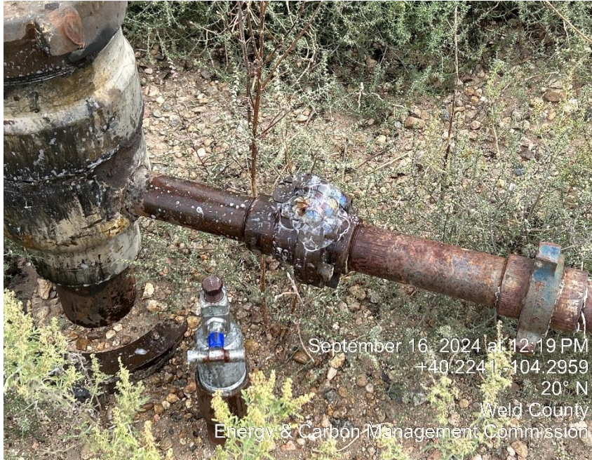
Balon appears to be leaking
