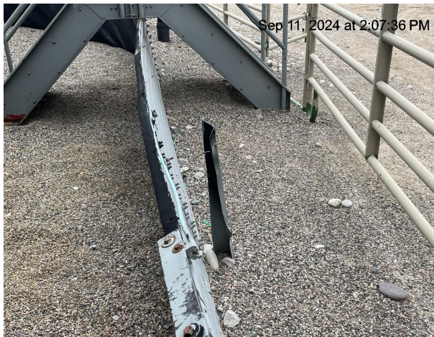
Photo # 9831 Secondary containment damaged/buckling
