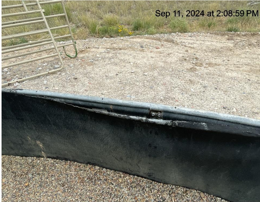
Photo # 9833 Secondary containment liner showing some signs of damage near top of containment ring
