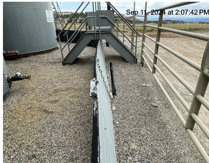
Photo # 9832 Secondary containment damaged/buckling
